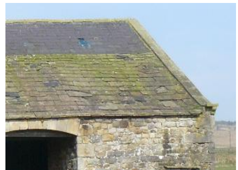
General condition of barn roof - east slope
