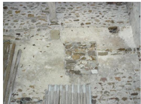
Infilled window to east elevation
