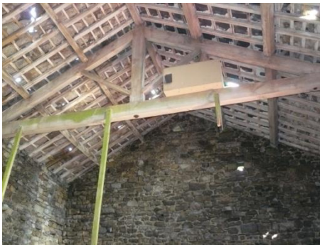
Barn roof - note truss in sound condition
