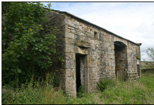
Entrance facade to barn
