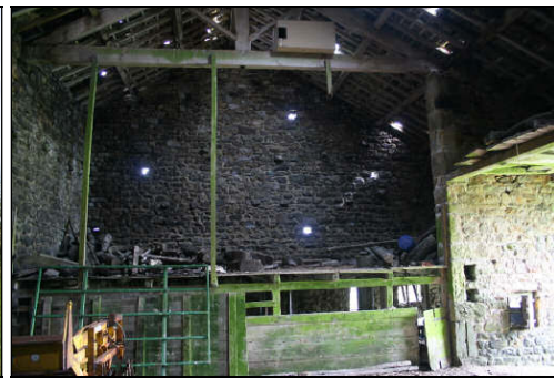
Barn interior with cart entrance to right
