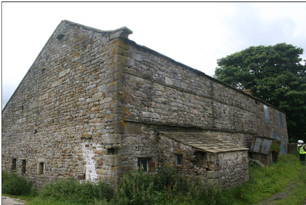
Front and side elevation to barn
