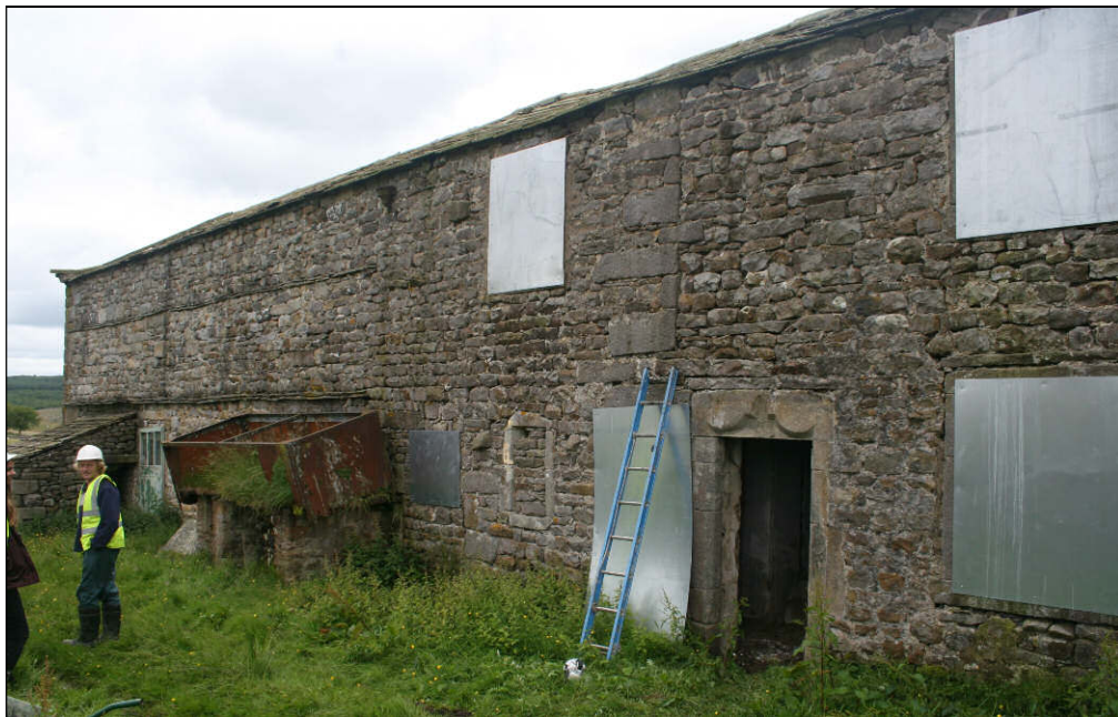
Front elevation, showing earliest phase to the left of present entrance to the house
