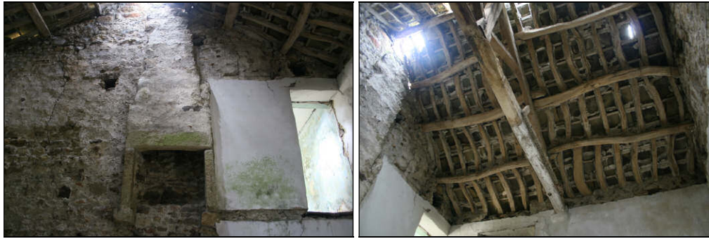
Interior of central unit showing first floor fireplace and roof
