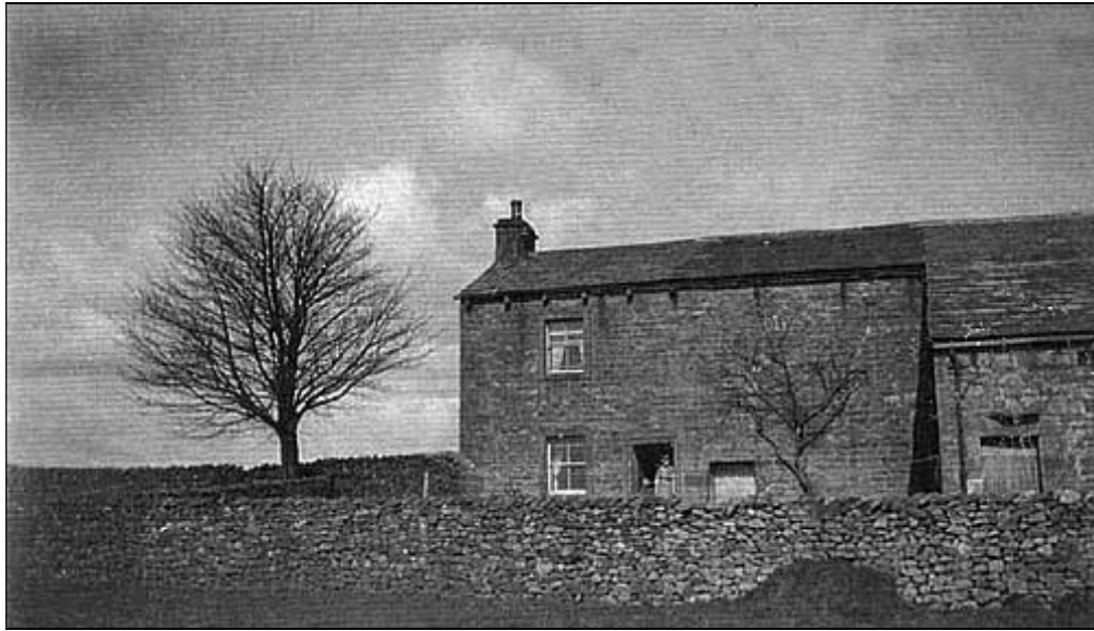
Photograph of rear elevation taken before closure of the farmhouse, possibly 1950s, from the late May Jackson collection ( www.dalehead.org/cocklick_end.htm )
