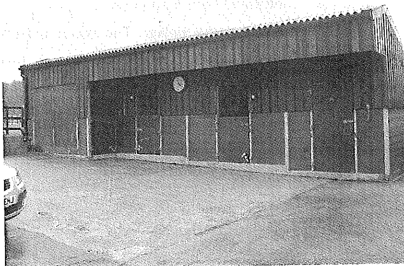
Stables to be retained.
