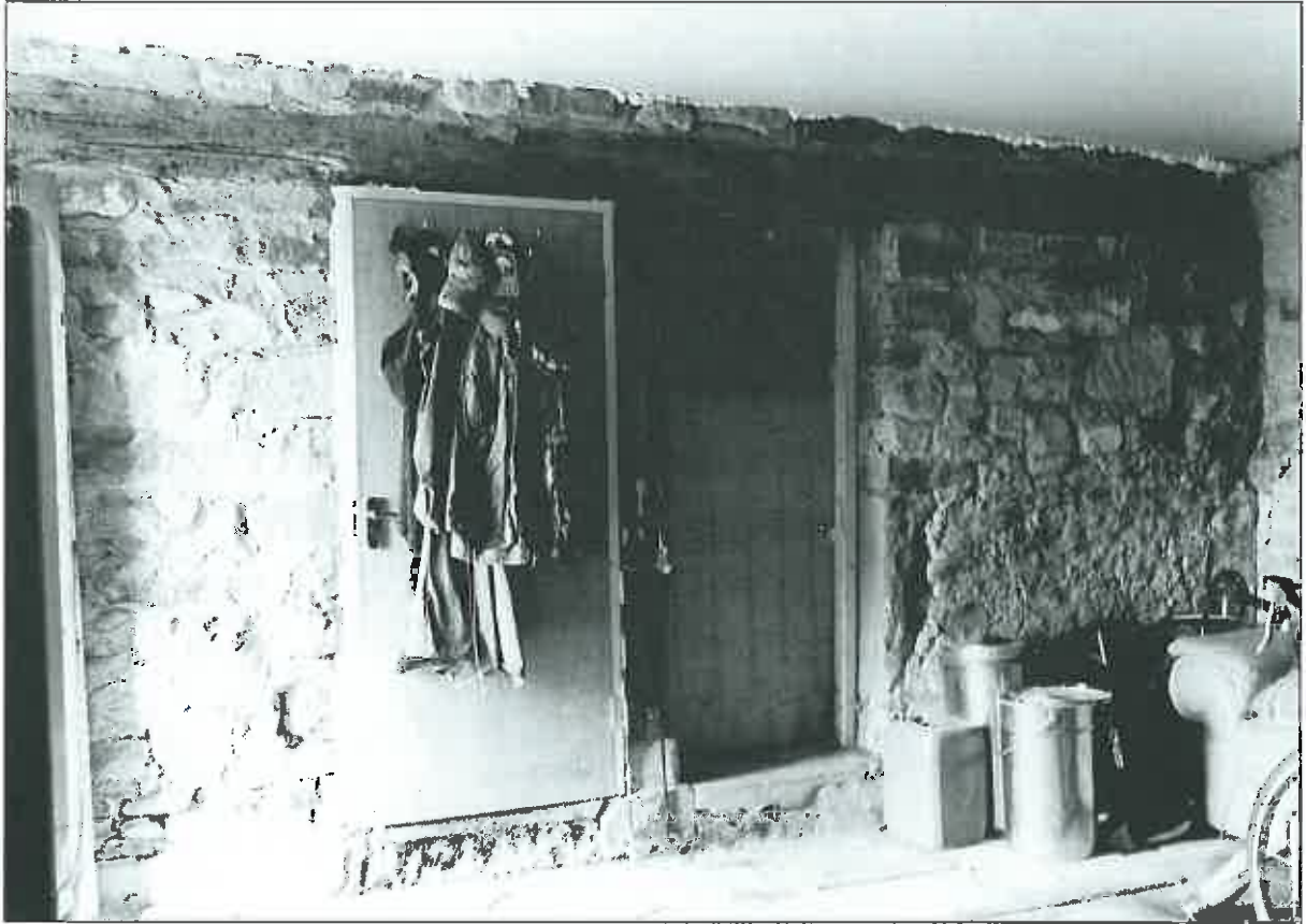
Photo 10: Remains of timber partition with pair of doorways, west side of housebody
