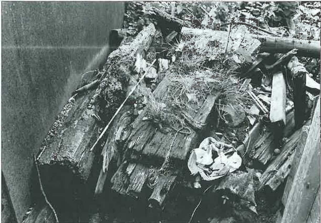
Photo 11: Remains of roof timbers from house, including likely base of upper cruck, presently in derelict outbuilding
