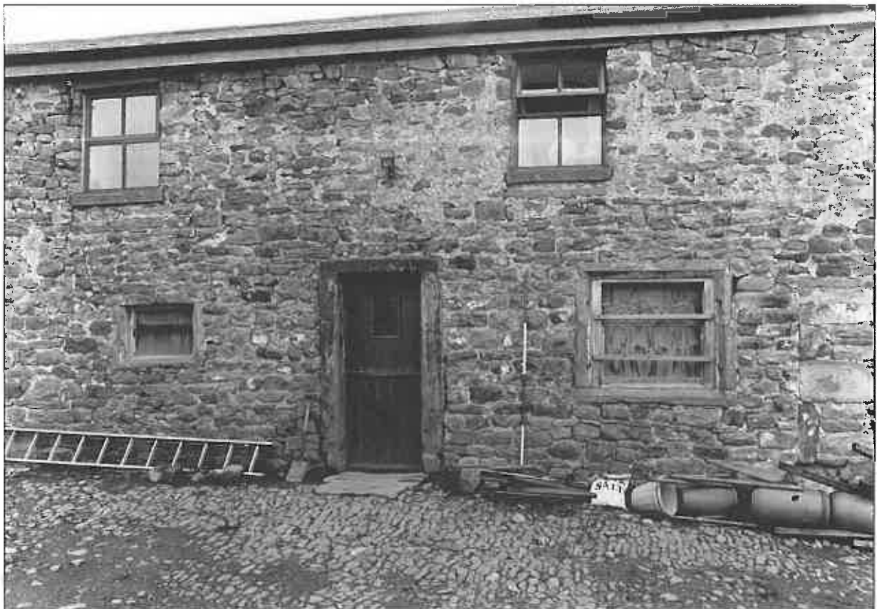
Photo 2: Front of the farmhouse (central part)
