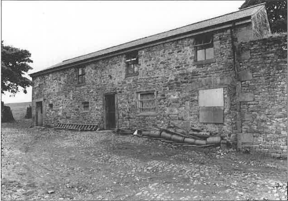
Photo 1: The front elevation of the farmhouse, from the south-east
