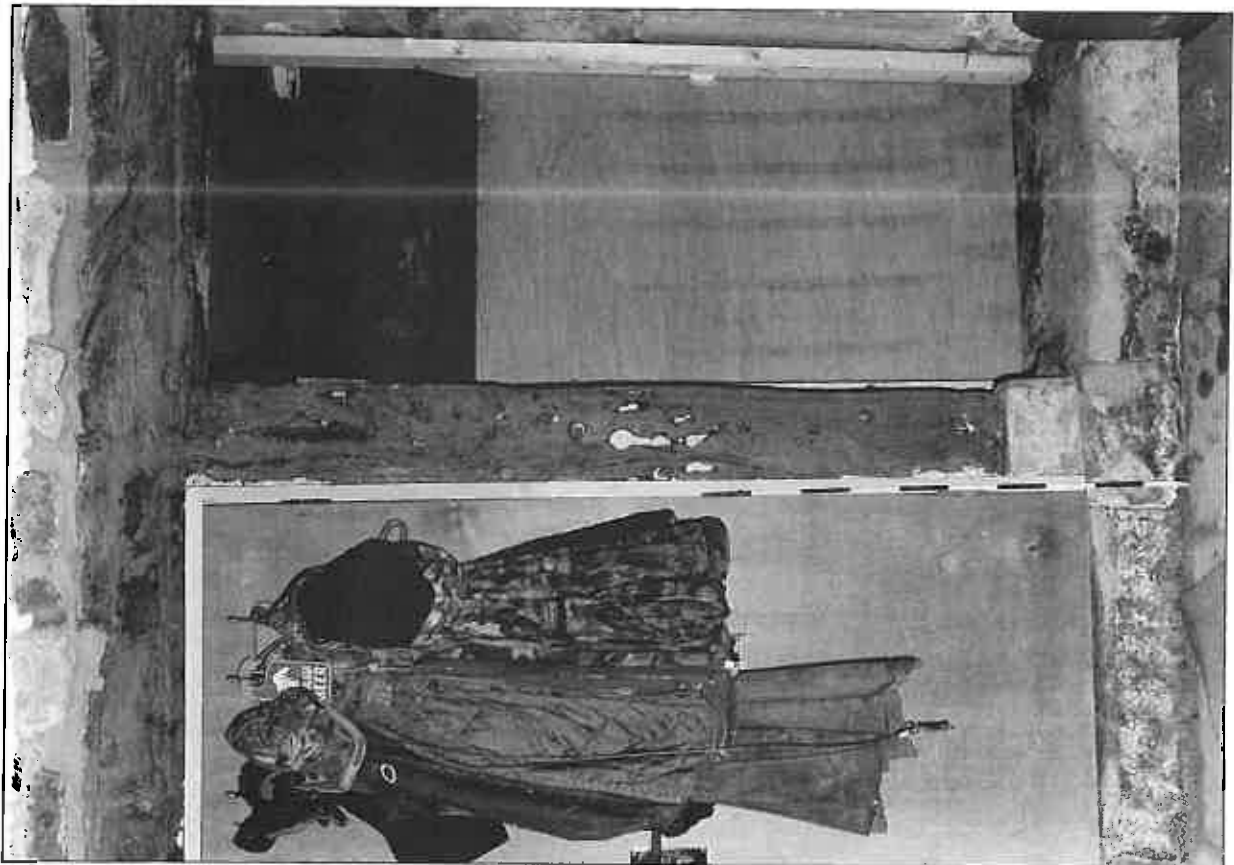
Photo 13: The stud between the pair of doorways, with pad-stone, west side of housebody
