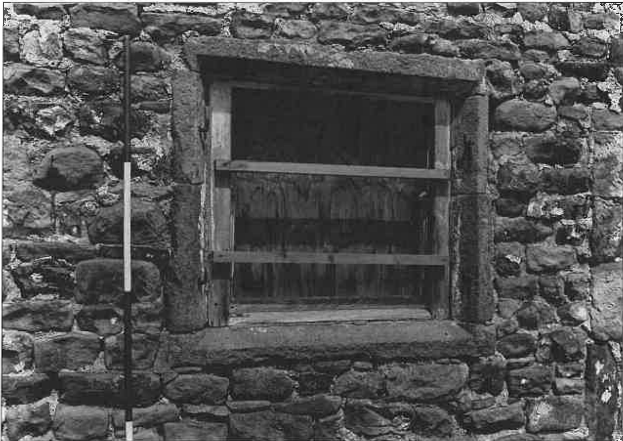
Photo 7: Detail of altered housebody window in south elevation
