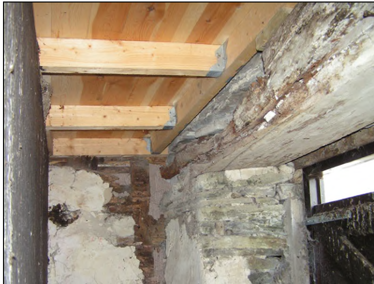
Indicative example of access point (rhs) and baffle to reduce light and air movement (lhs)
