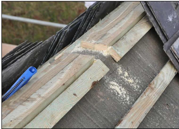
Battens be cut beneath the ridge to enable bats to access to both sides of the roof, but without access to roof void
