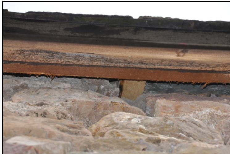
Indicative example of fascia board with bat access gap beneath
