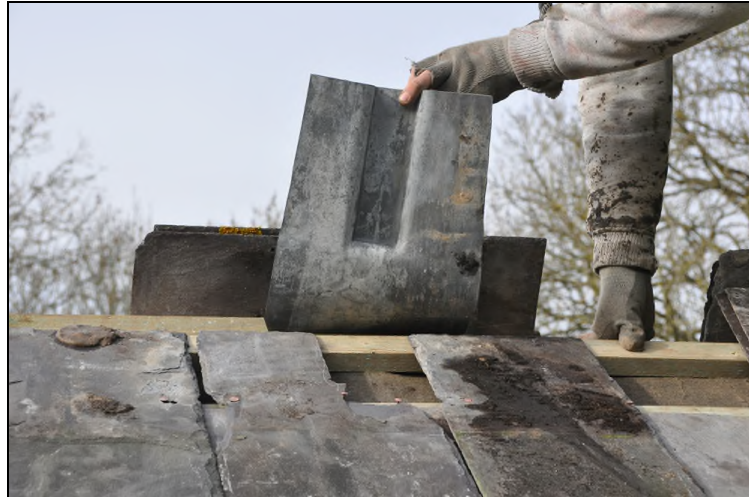
Indicative example of lead saddle associated with ridge access
