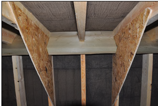
Ridge exposed between baffles
