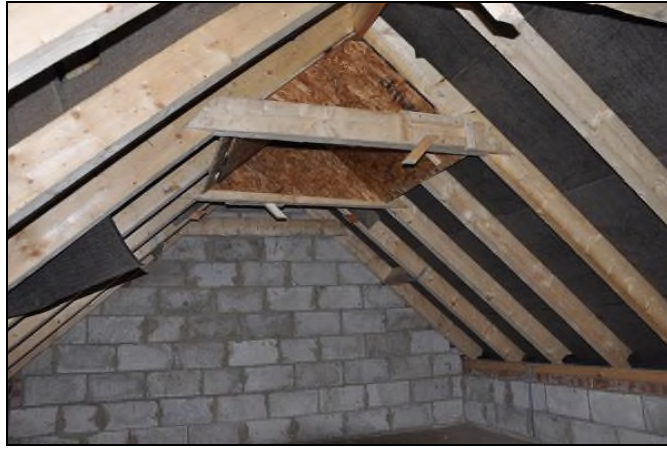
Example of baffles in a roof void
