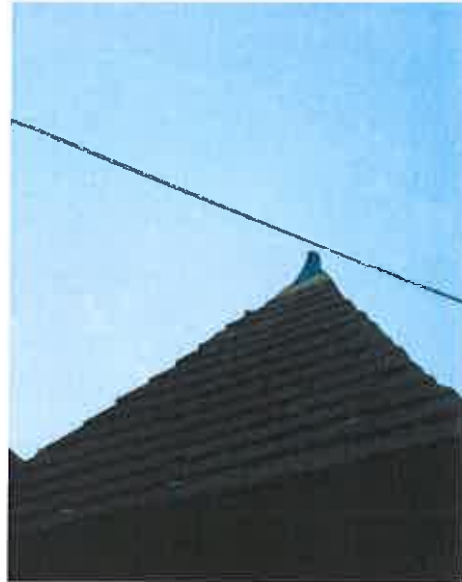
Lead flashing on eastern wing of main building showing obstruction by foam.
