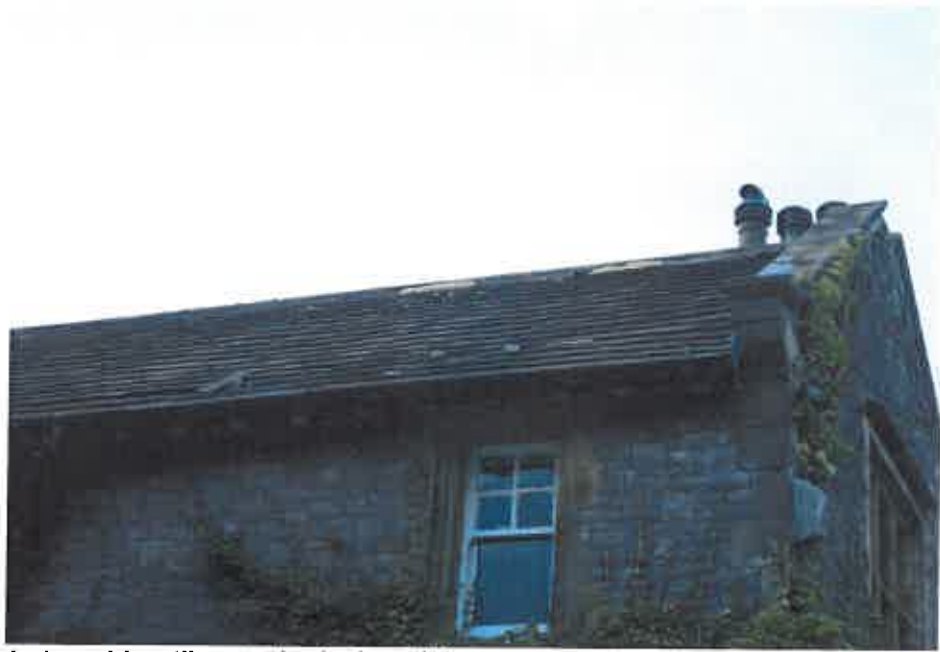
Gaps below ridge tiles and missing slates.
