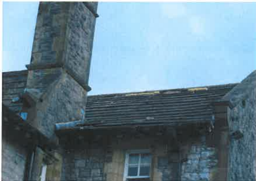
Gaps below ridge tiles suitable for roosting bats
