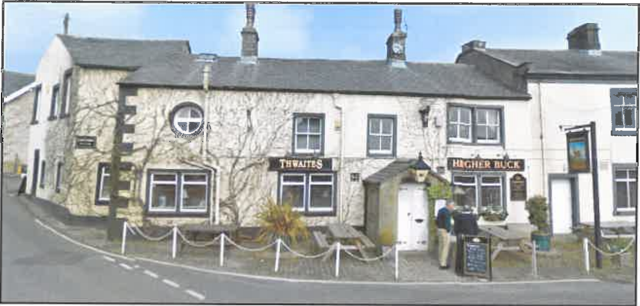
Figure 2. The southern elevation fronting the Square with adjoining houses to the right
