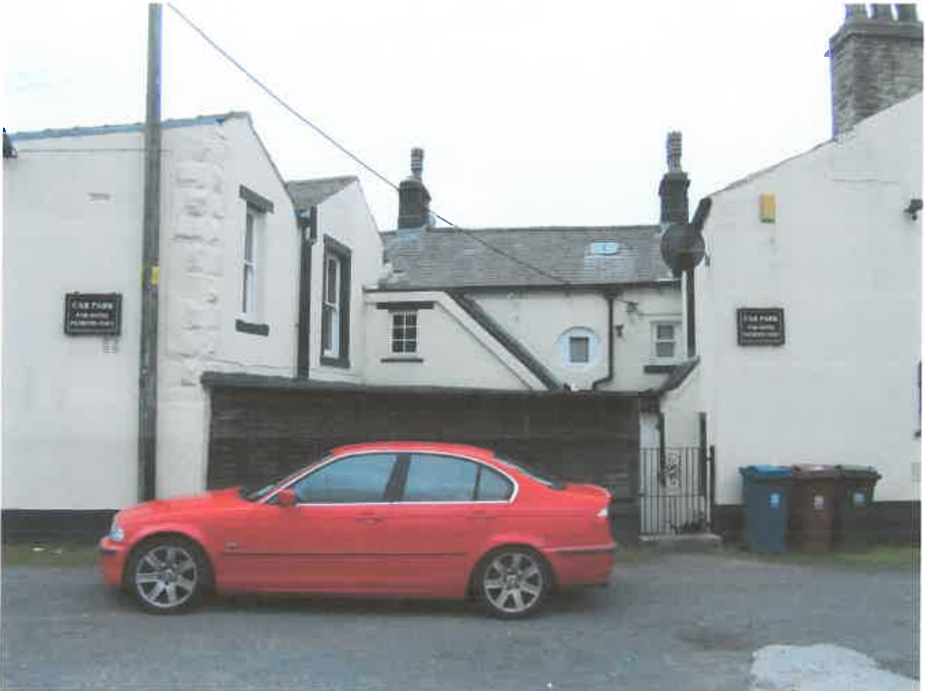
Figure 4. Rear elevations from the car park, main part. The wooden fence to the centre conceals an external fridge. This is to be replaced with a more attractive rendered masonry enclosure which will blend with the adjacent walls.
