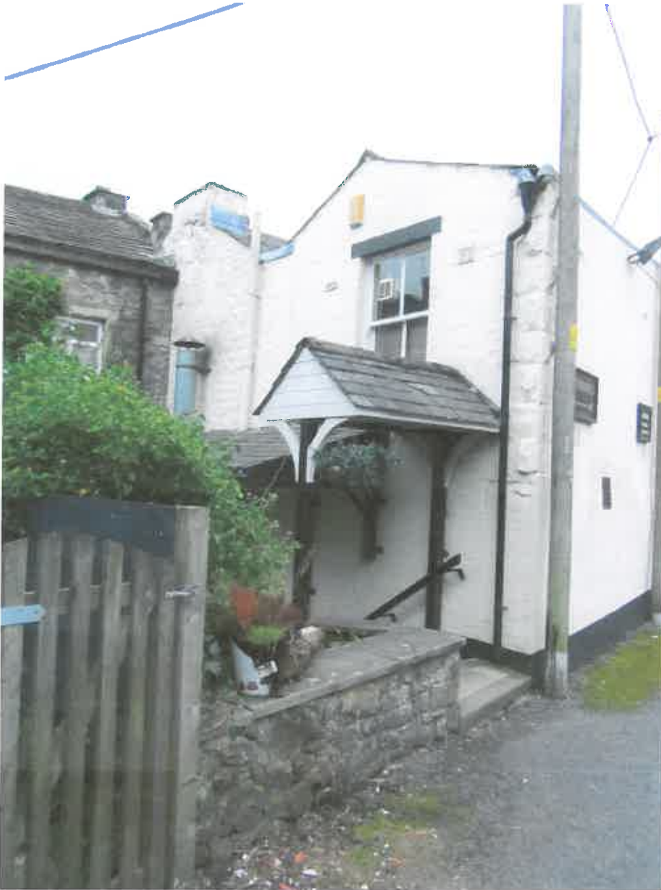
Figure 11. Boundary to the rear of what was number 77, where a wider entrance is to be formed
