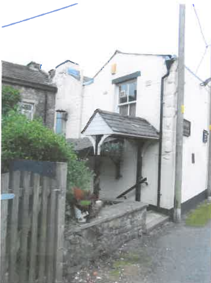
Figure 3. Rear entrance and boundary from the carpark. The canopy is to be removed and the low wall adjacent taken down. Neither are original features.
