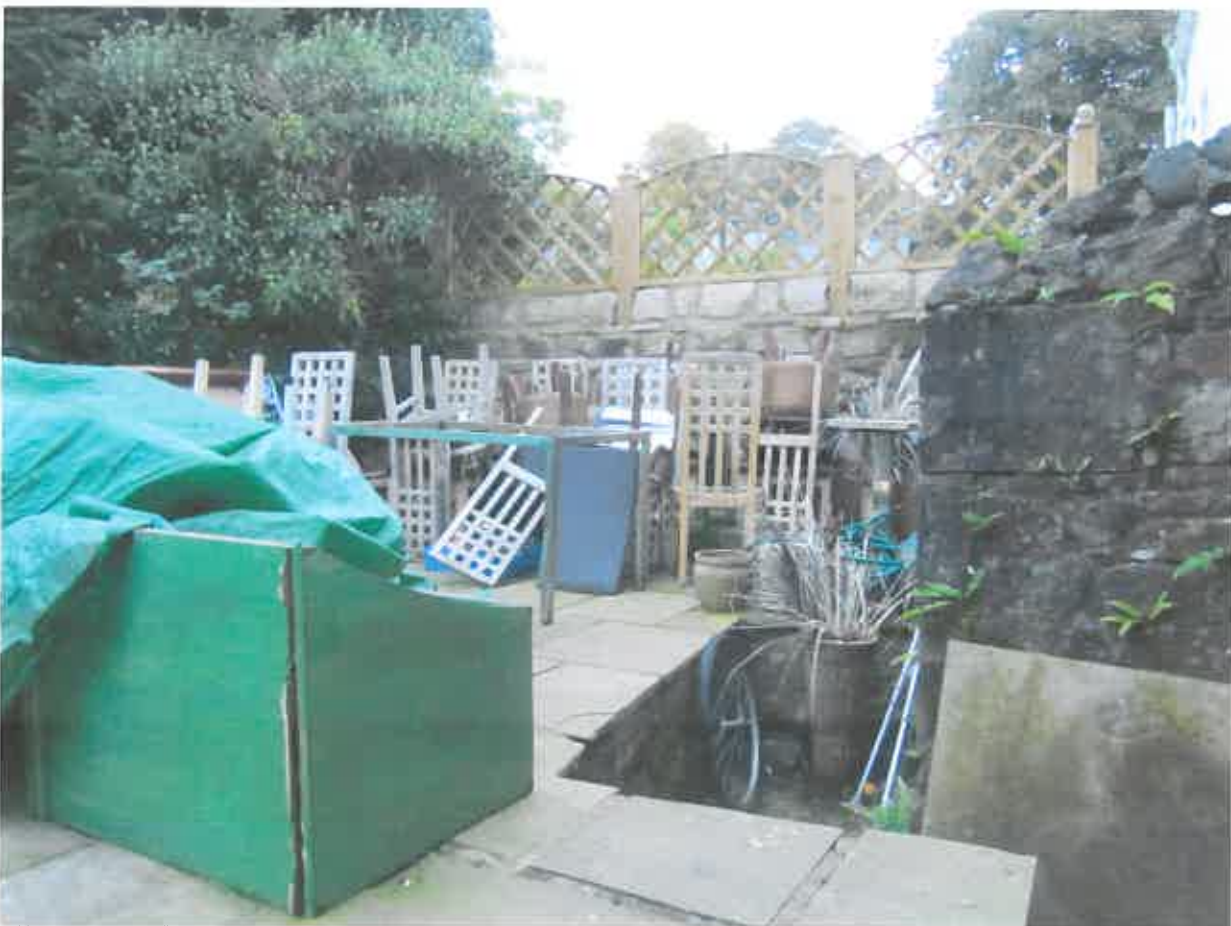
Figure 10. Yard altered as beer terrace to the rear of what was number 76 with rebuilt garden wall and fencing.
