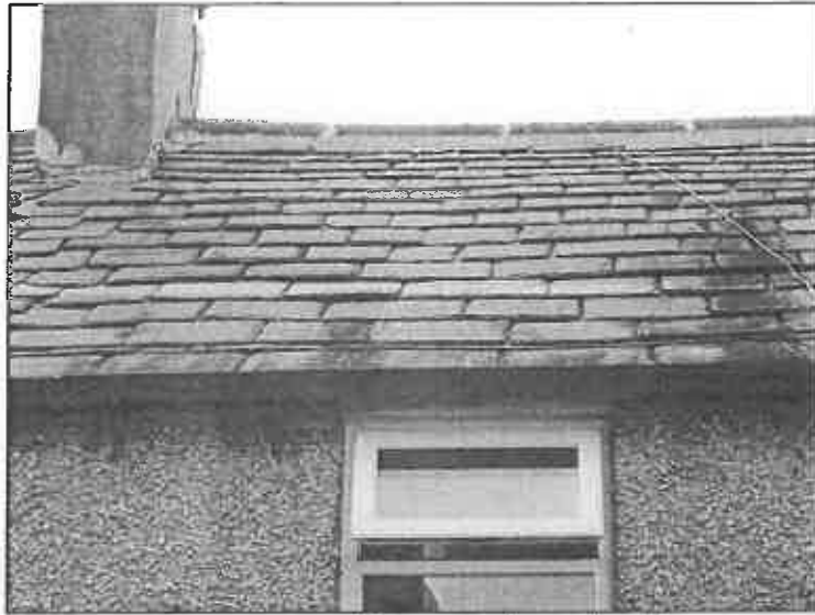
Figure 5: Gaps in slates on southern elevation.
