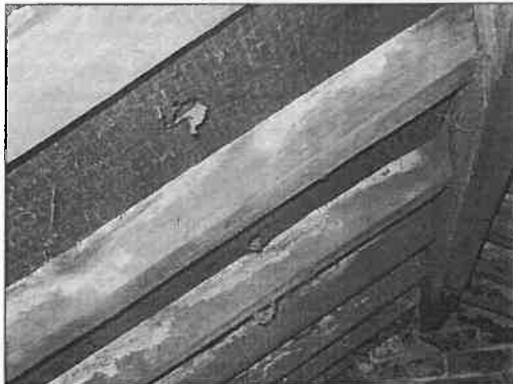
Figure 6: Southern elevation interior – example of holes cut in felt lining to complete thorough endoscope inspection, no evidence found.
