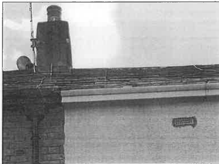
Figure 2: Gaps in slates – suitable roosting features that have been retained (northern elevation).
