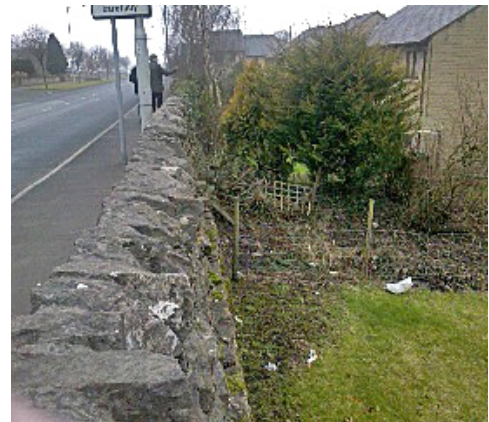
Fig 9: View along Chatburn Road with the Kiln Close development on the right.
