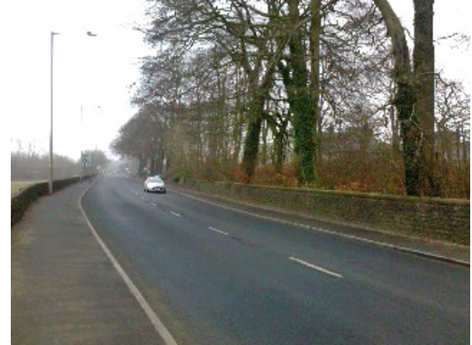
Fig 5: View along Chatburn Road looking north eastwards with application site on left. Note the strong directional emphasis created by road, footpath and stone walls.
