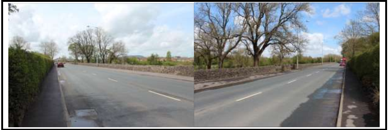
View to exiting access point
