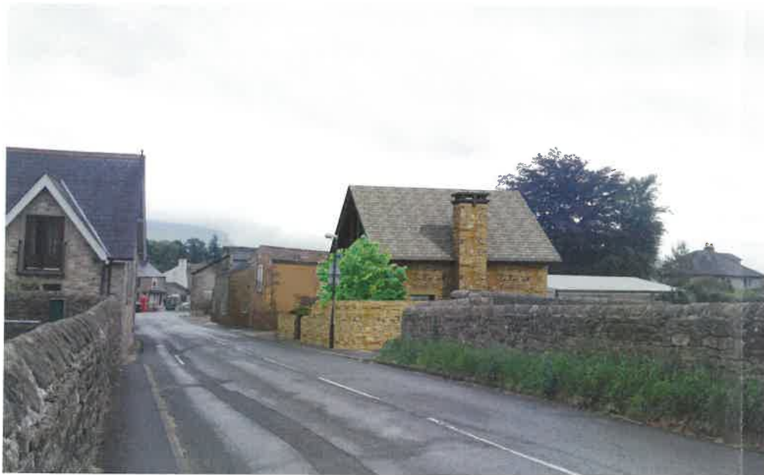
PERSPECTIVE LOOKING DOWN FELL ROAD INTO WADDINGTON
