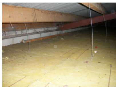
Fig 9: roof void building 'B'
