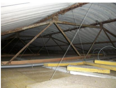
Fig 8: roof void building 'A'
