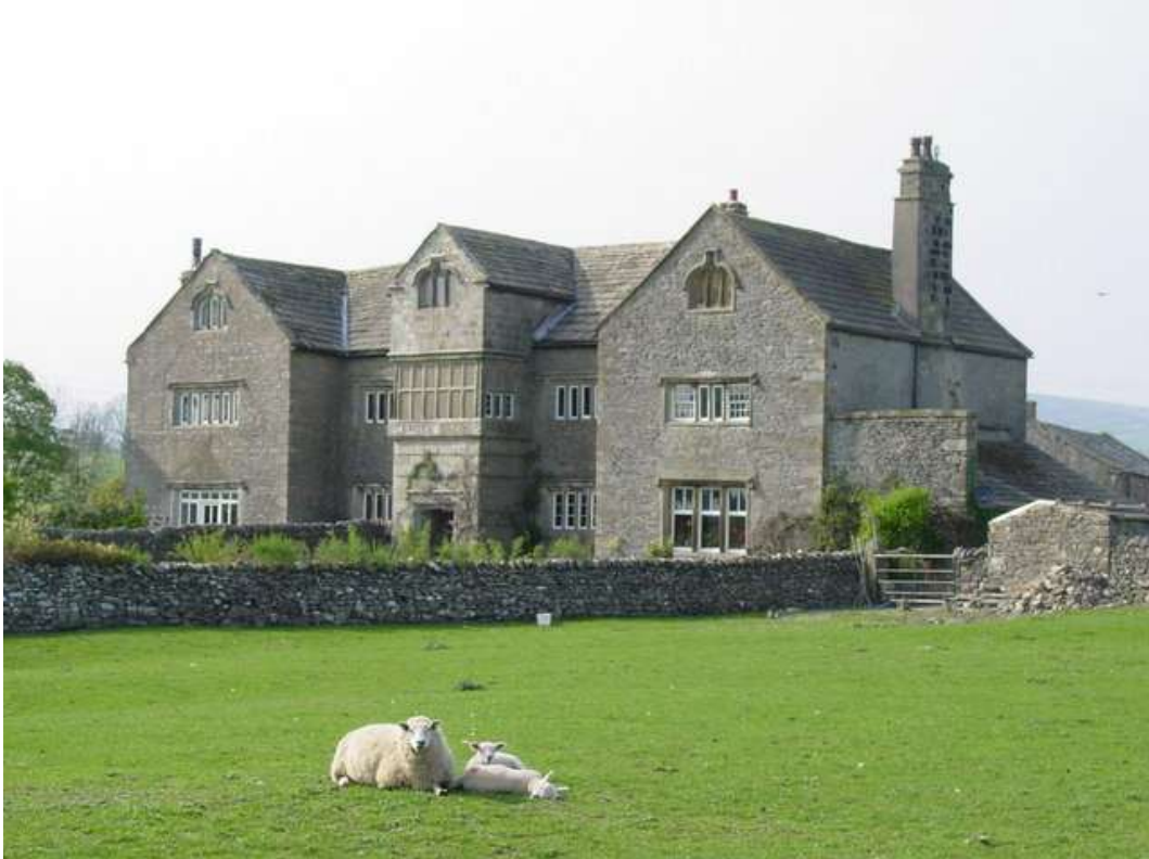
Photo G – Hammerton Hall, Slaidburn
