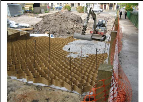
Appropriate aggregates are back filled filling all of the cells
