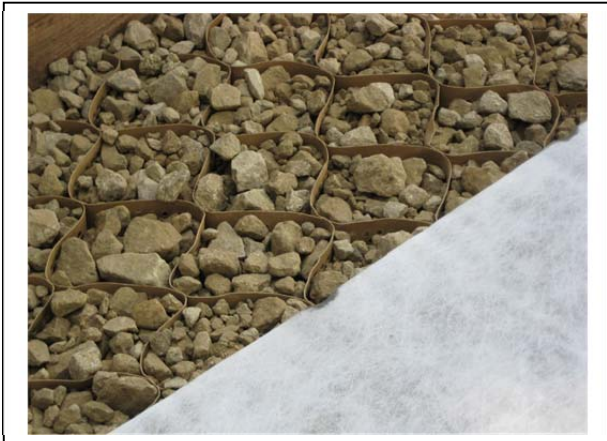
Geotextile fabric laid over filled cells then covered with temporary / permanent wearing course as per construction specifications
