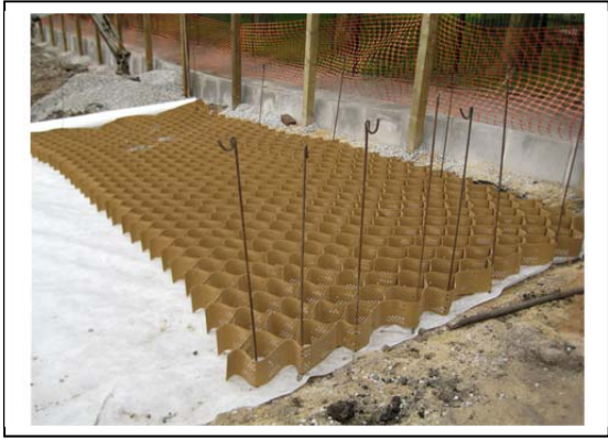
Laying of geotextile fabric with the cellular confinement system pined in place
