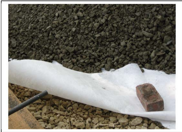
Geotextile fabric laid over filled cells then covered with temporary / permanent wearing course as per construction specifications
