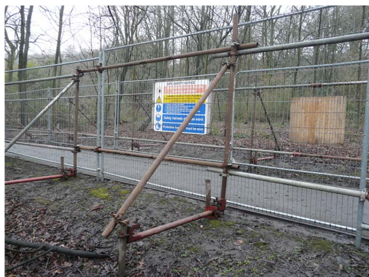
Example of scaffold framework with 'Heras' fencing attached
