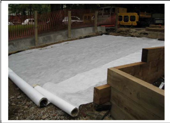
Laying of geotextile fabric with the cellular confinement system pined in place
