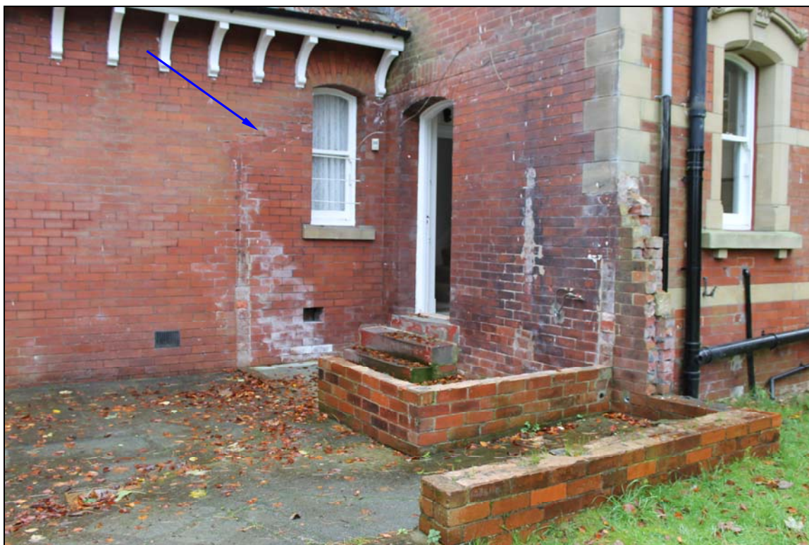
13. Detail of the rear, showing evidence of porch or canopy with single-pitch roof (indicated)
