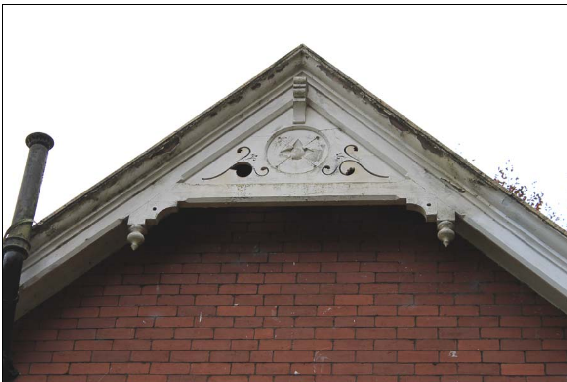
14. Timber bargeboards with pendants on the north gable
