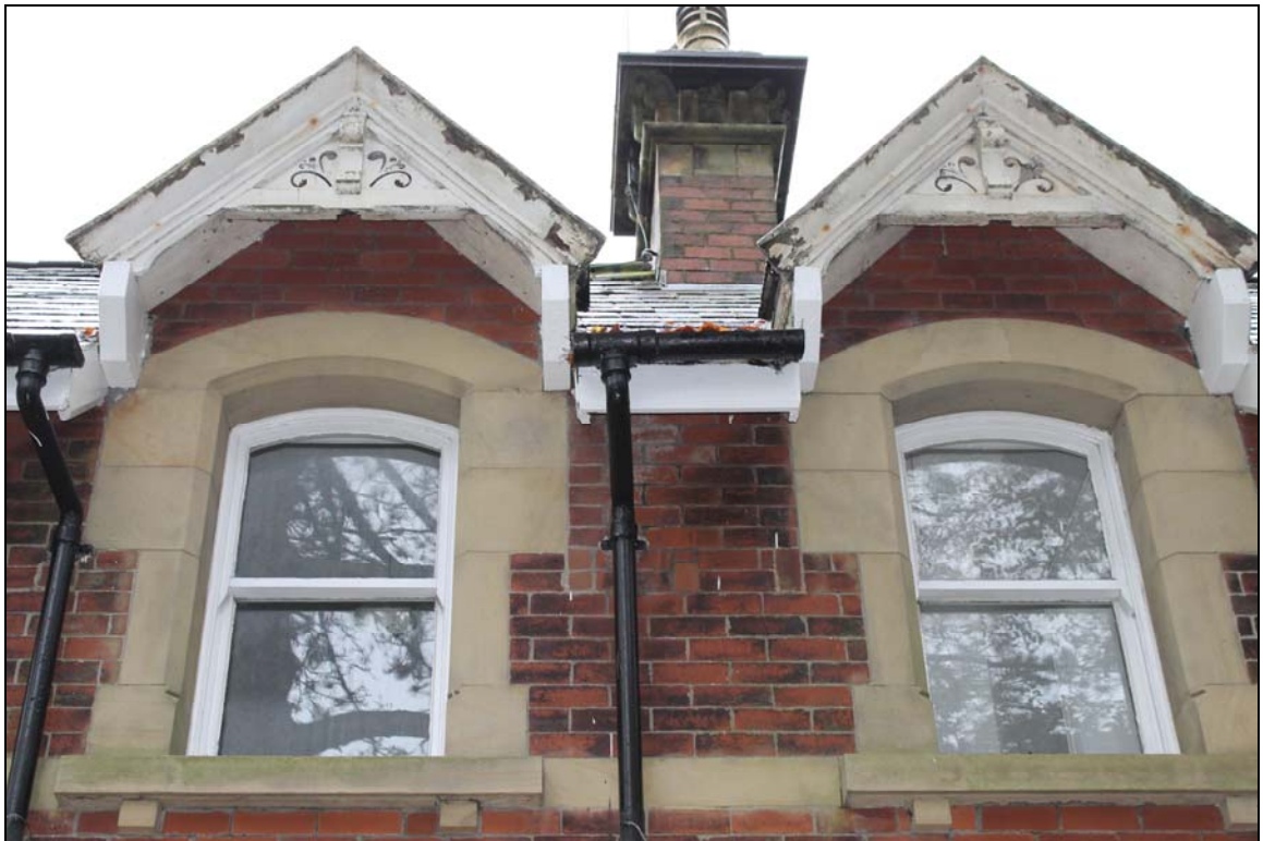
10. Timber bargeboards of first floor windows on west elevation; the windows lack labels
