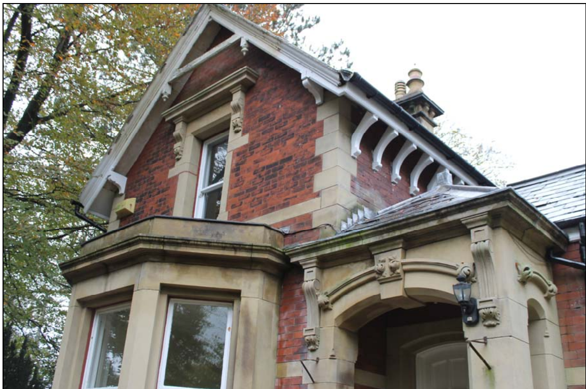
7. Typical Italianate details include the wide bracketed eaves and chimney caps
