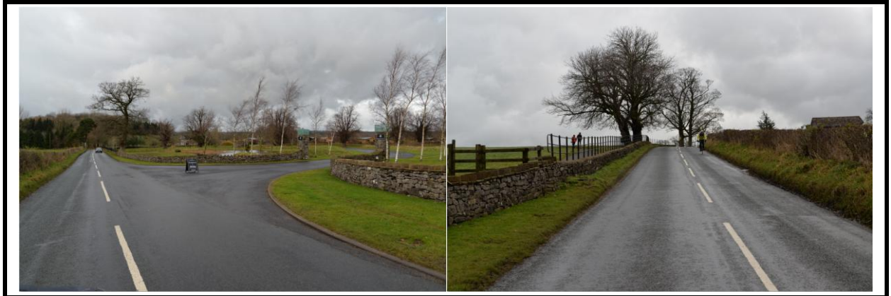
View of existing leisure site access point and uphill incline.
