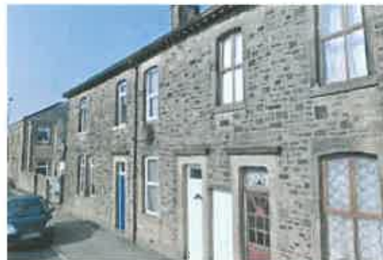
Existing development of Crumpax Avenue
