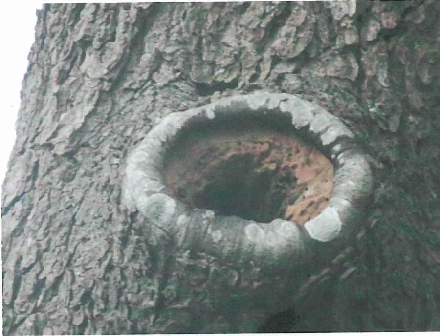
Plate 5: Example of potential bat roost feature (T22) present within the site
