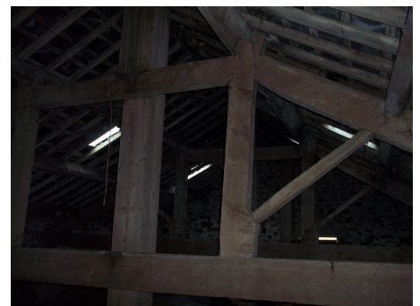
Figure 6: roof in loft
