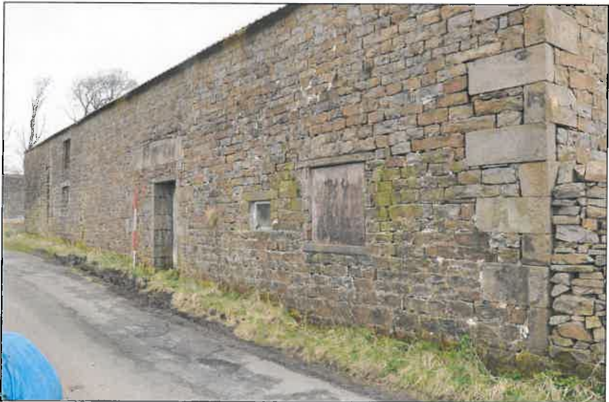
Photo 11: West elevation of main part of barn, from the south-west
