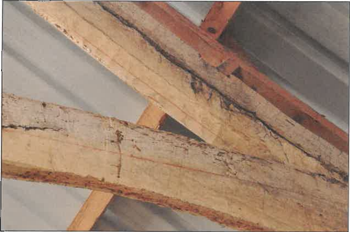
Photo 30: Truss III: detail of chalk line and tooling marks, east end, from the south
