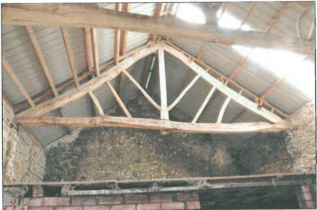
Photo 25: South truss in barn (number 1), from the north
