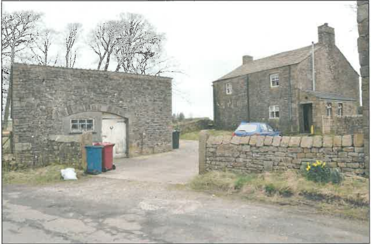
Photo 46: Trap house and rear of farmhouse, from the south-west
