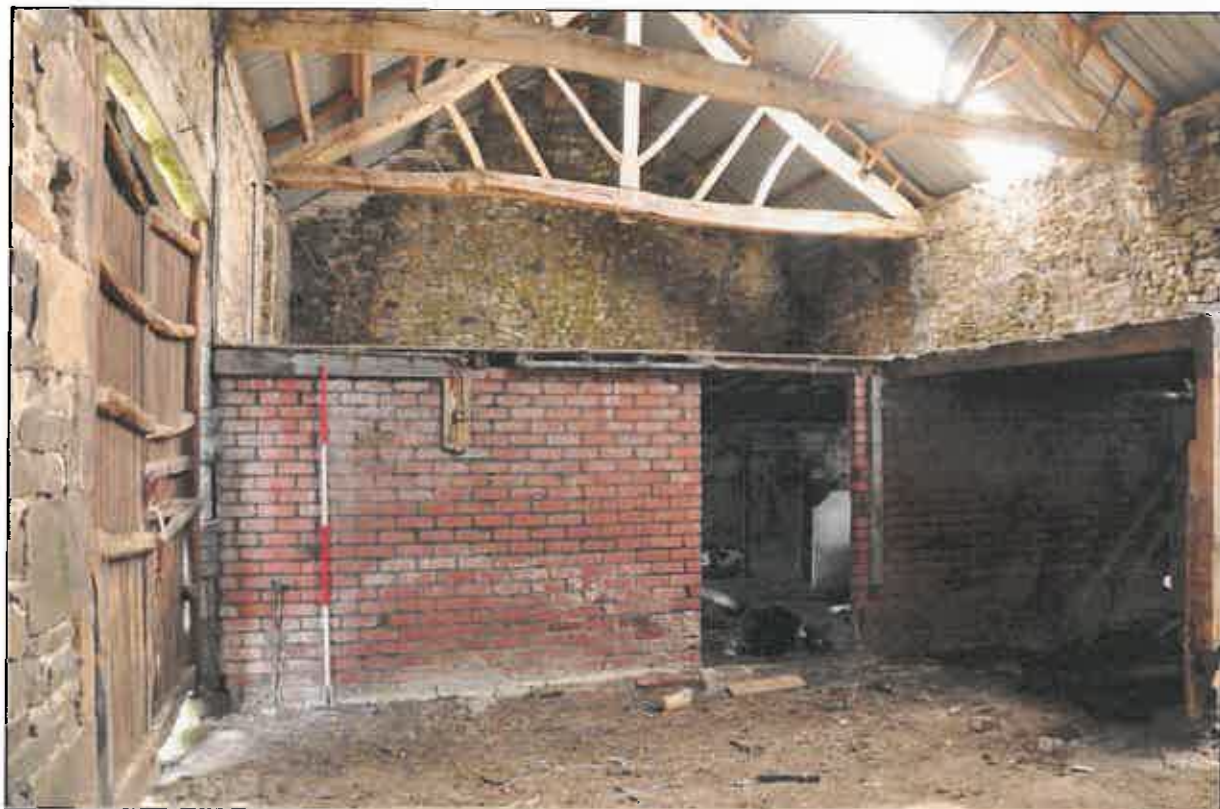
Photo 19: Interior of barn: brick wall enclosing shippon in south end
