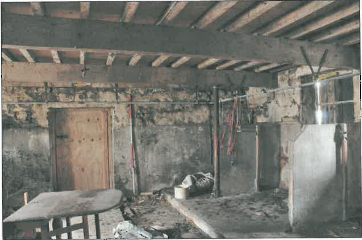
Photo 21: Interior of barn: modern shippon in south end, from the north-east
