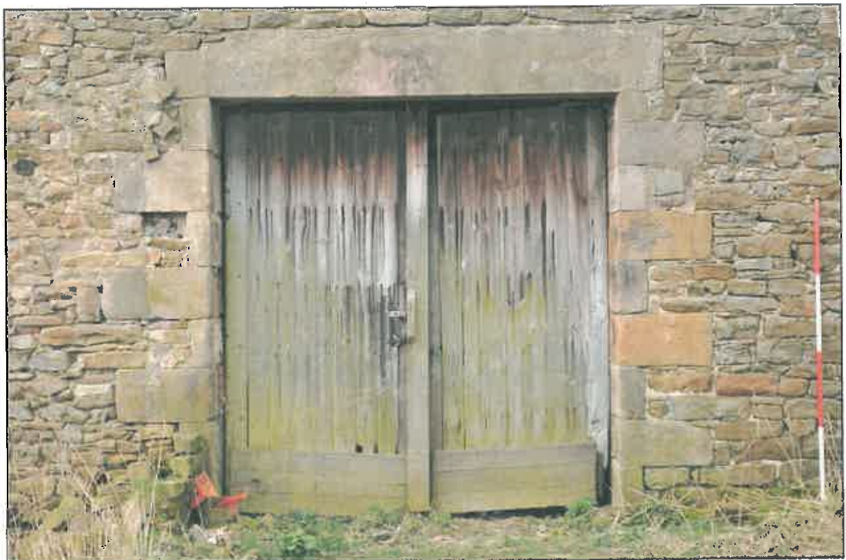
Photo 3: Cart entrance in east side of barn
