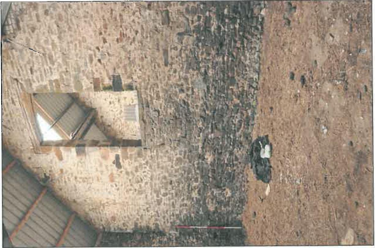
Photo 16: Interior of barn: cross-wall, from the south-east
