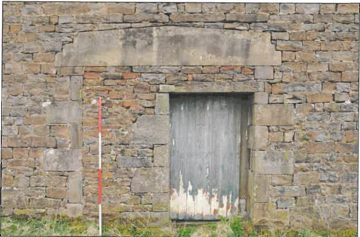
Photo 5: Cart entrance in west side of barn
