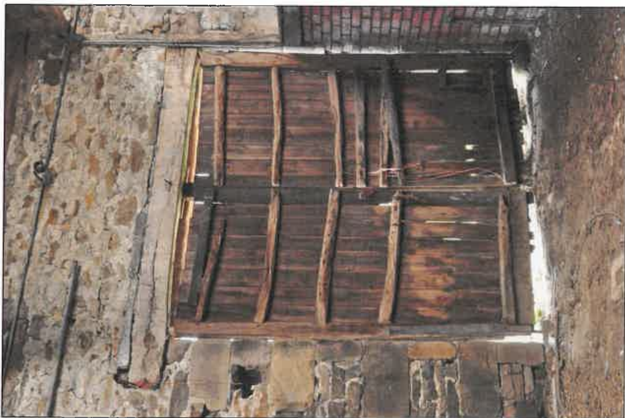
Photo 17: Interior view of doors in east cart entrance
