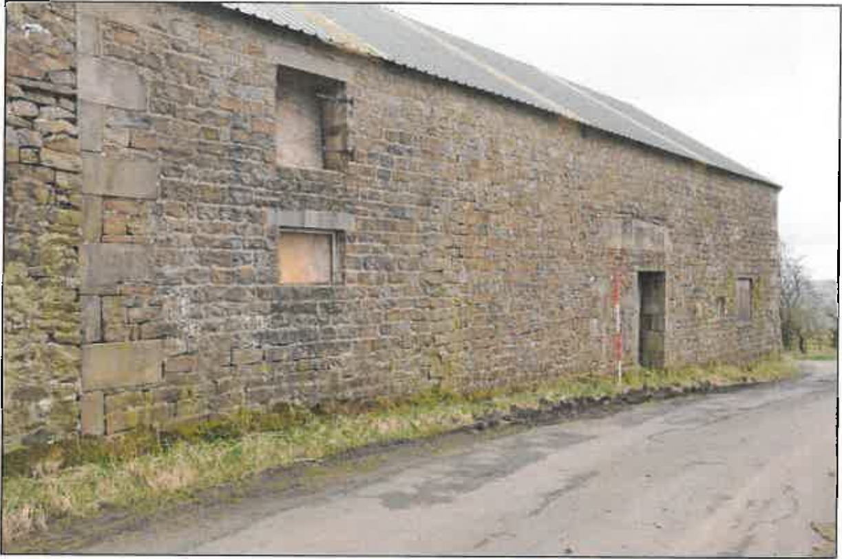
Photo 10: West elevation of main part of barn, from the north-west
