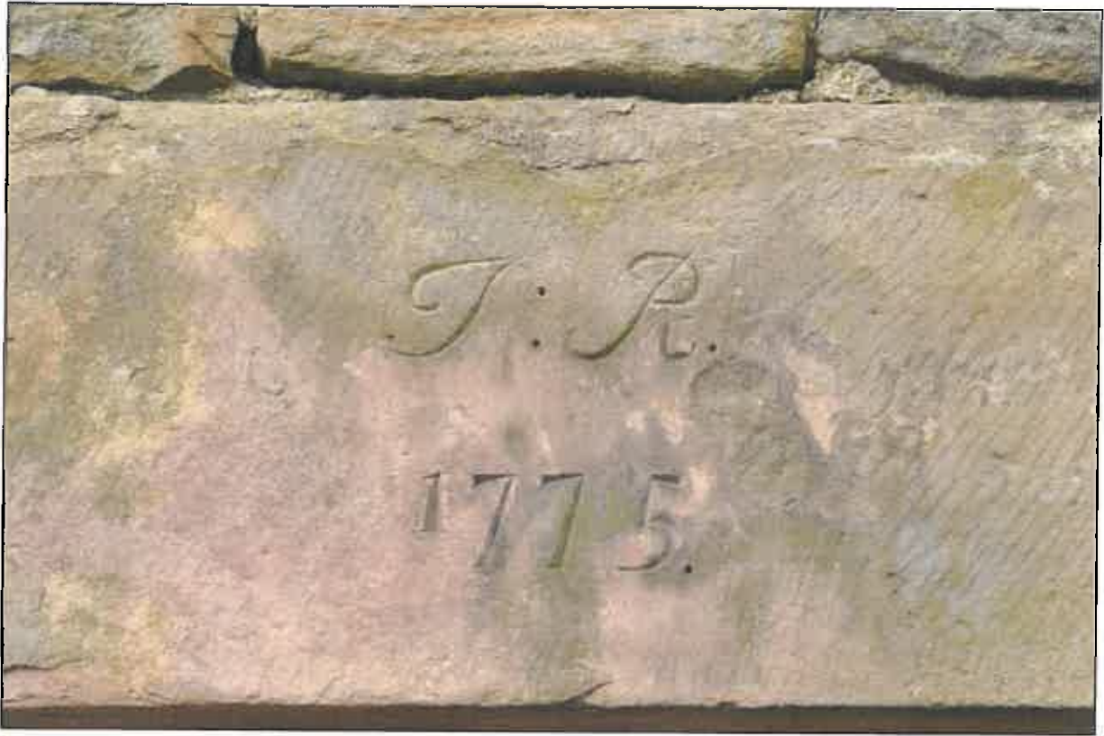
Photo 4: Detail of initials TR and date 1775 over east cart entrance
