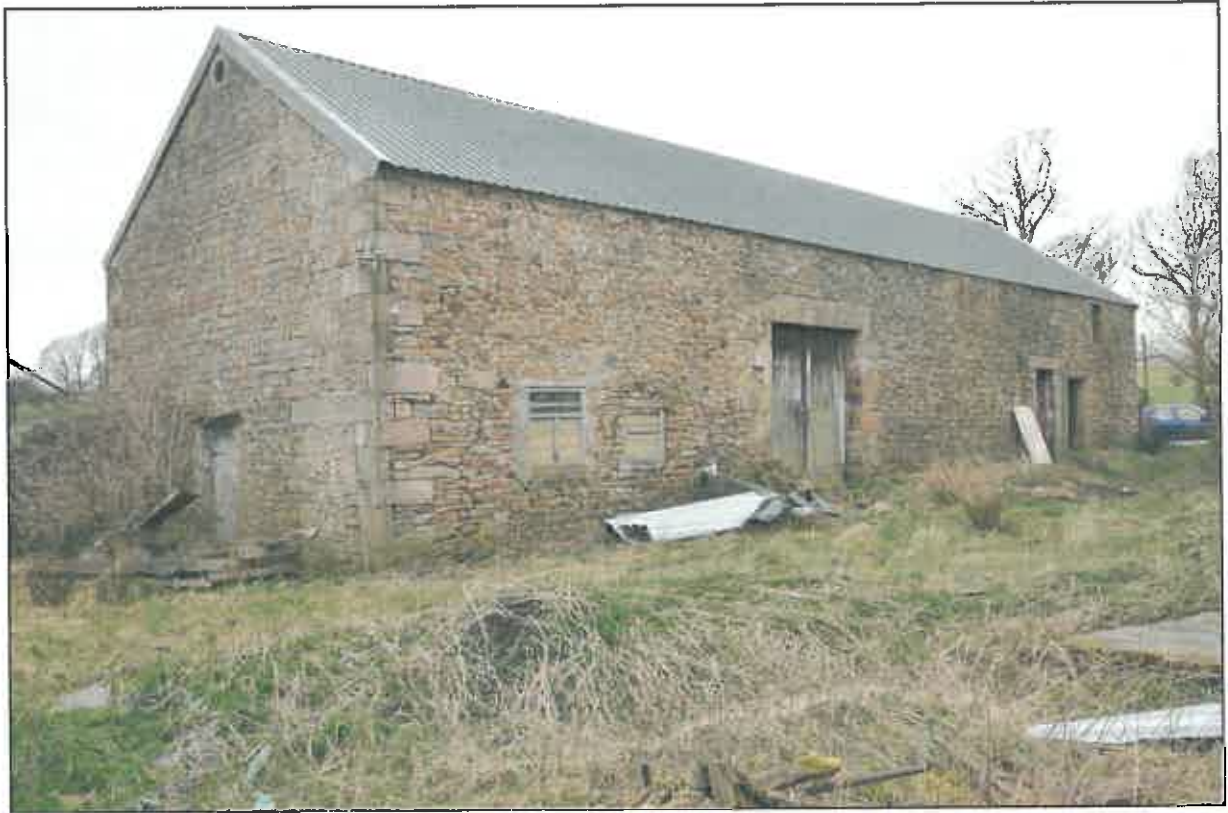
Photo 1: General view of the barn, from the south-east
