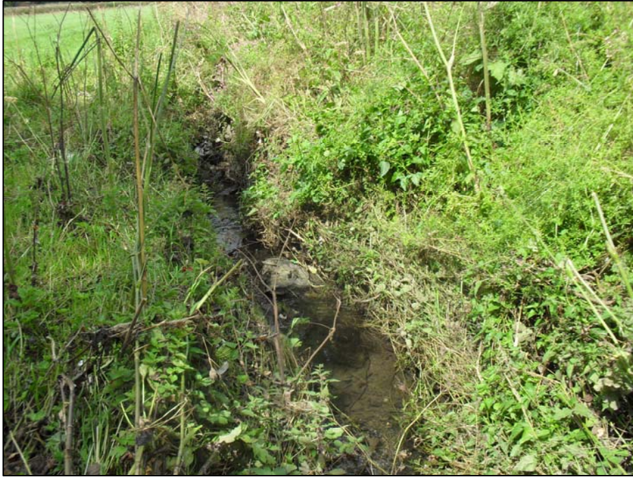
Plates 5. Watercourse channel with debris.
