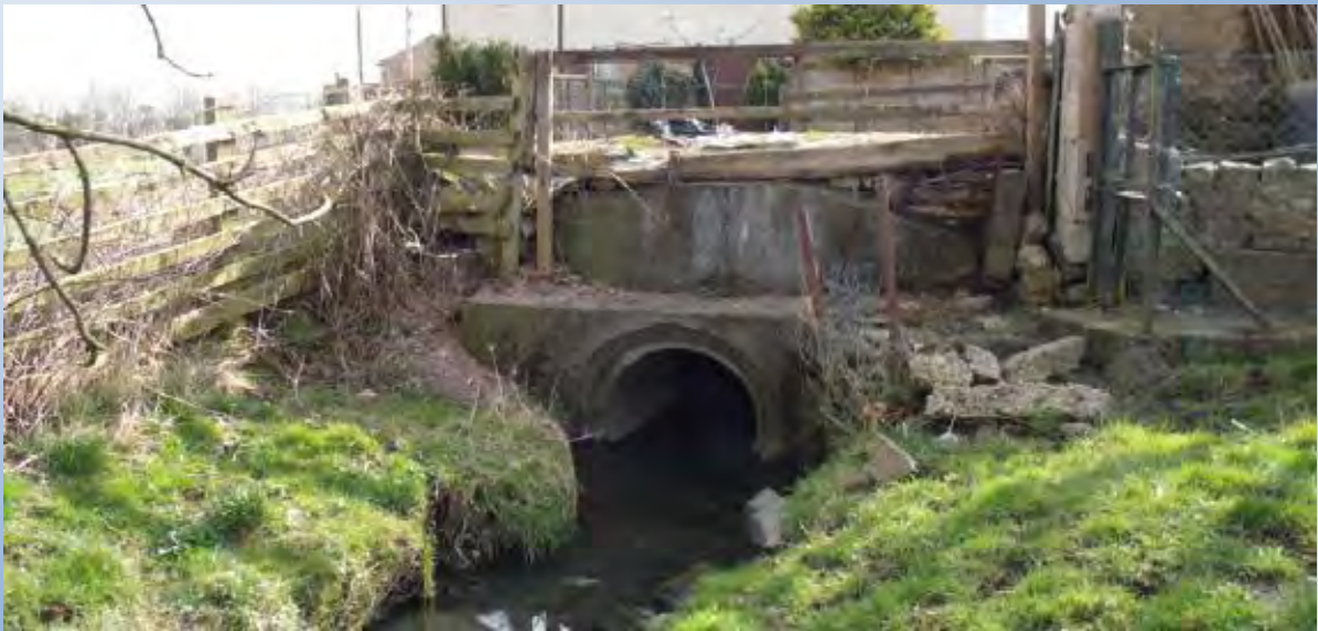
Figure 4: Photograph of Culvert Outfall along the South-Eastern Boundary.
