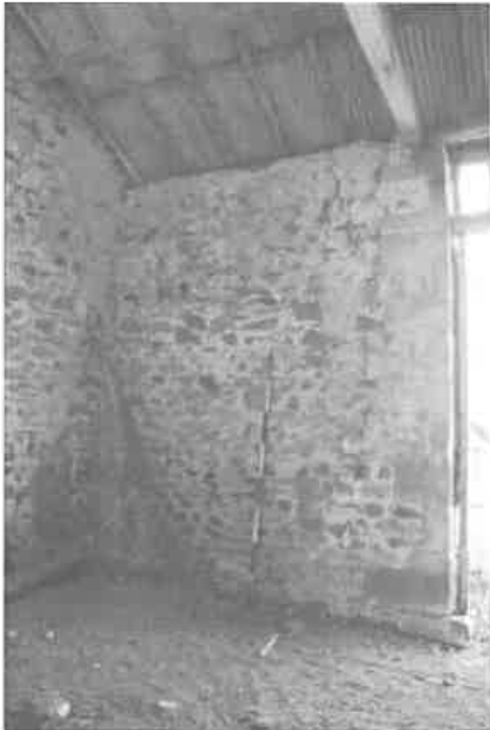
Figure 35 The cart entrance, showing the internal quoins
