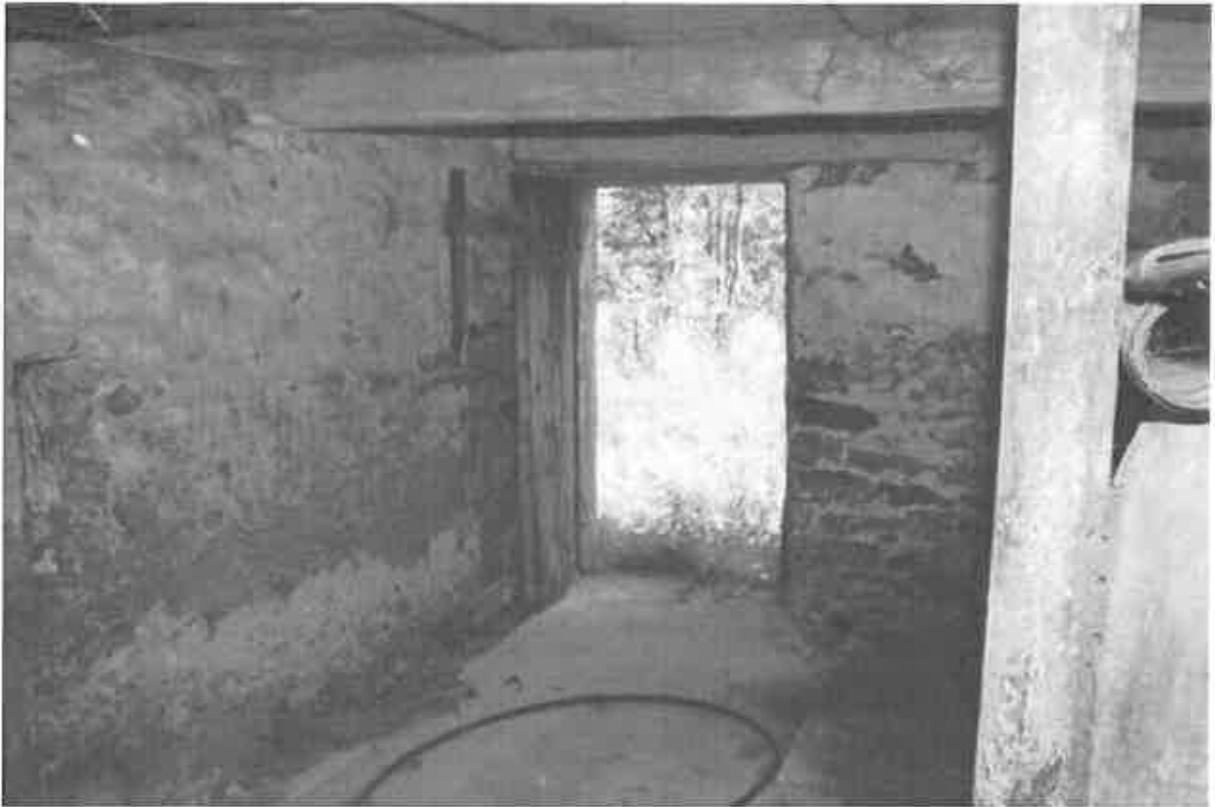
57 The doorway to the south east corner of the gable, showing the rebated door jambs and the door opening against the outer wall.
