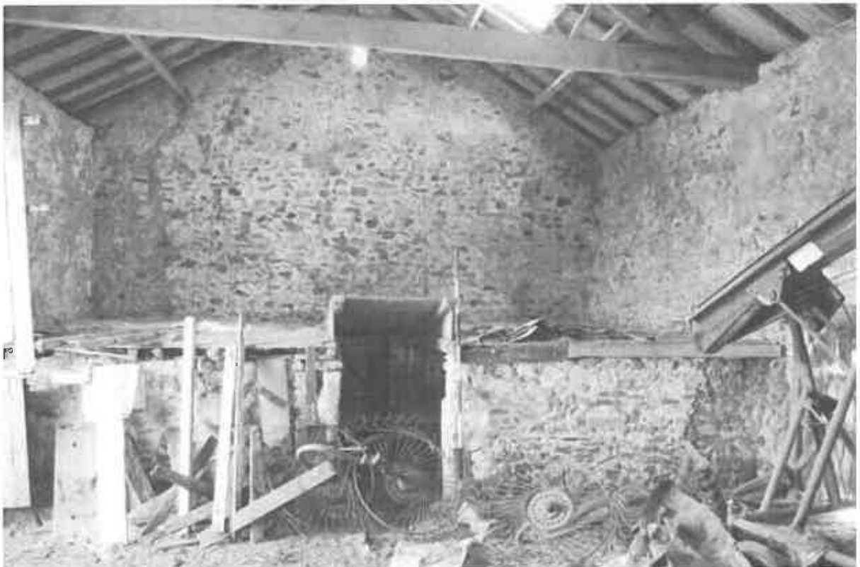
46 The south east gable and the internal partition
