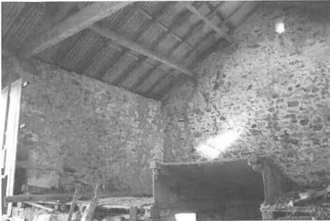
Figure 36 The north east internal elevation, showing the cart entrance and remainder of the elevation.
