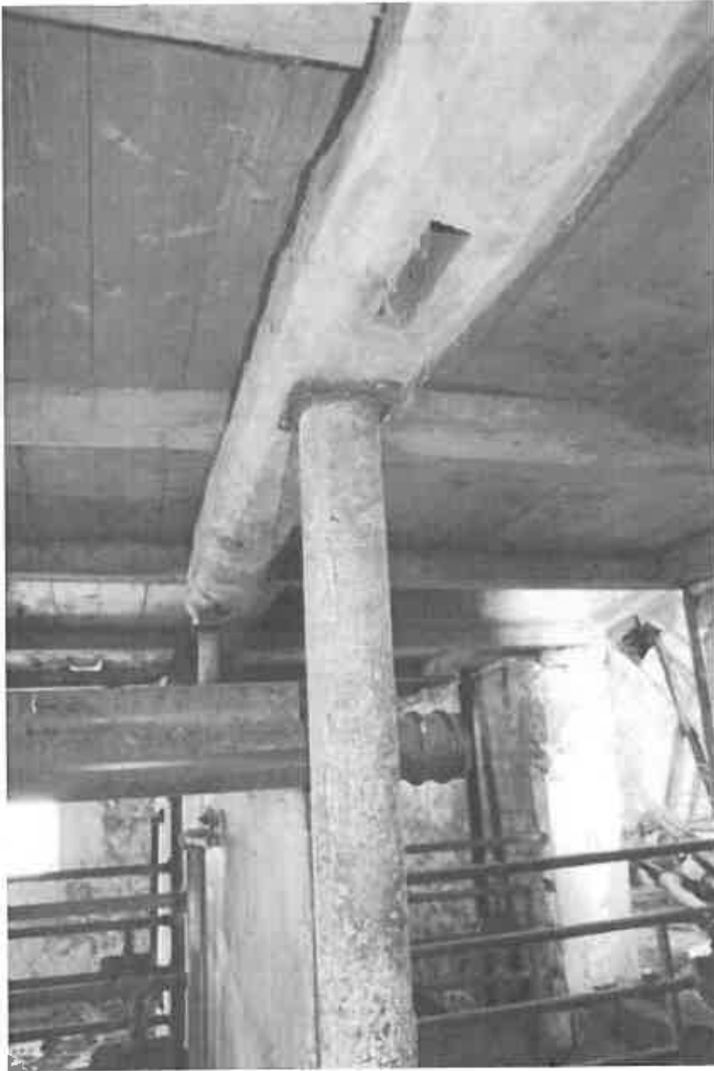
60 A notch to the underside of the floor beams.
