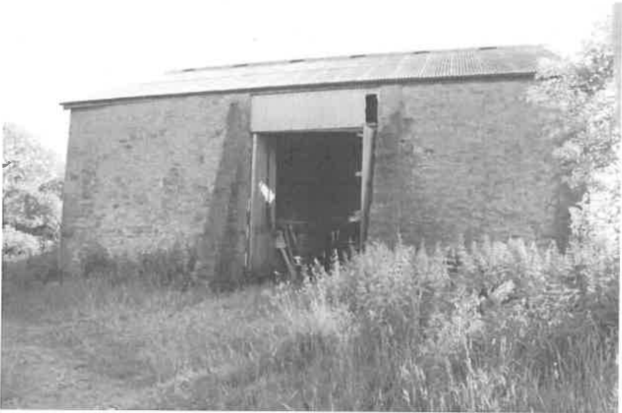
1 The north east elevation showing the cart entrance and butresses
