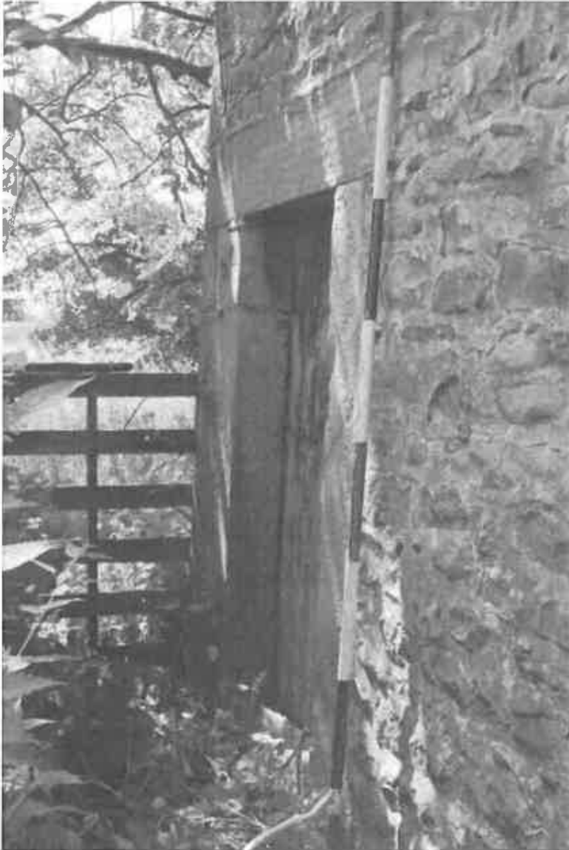
15 The left hand doorway to the south east elevation, showing the stone jamb/reveal.
