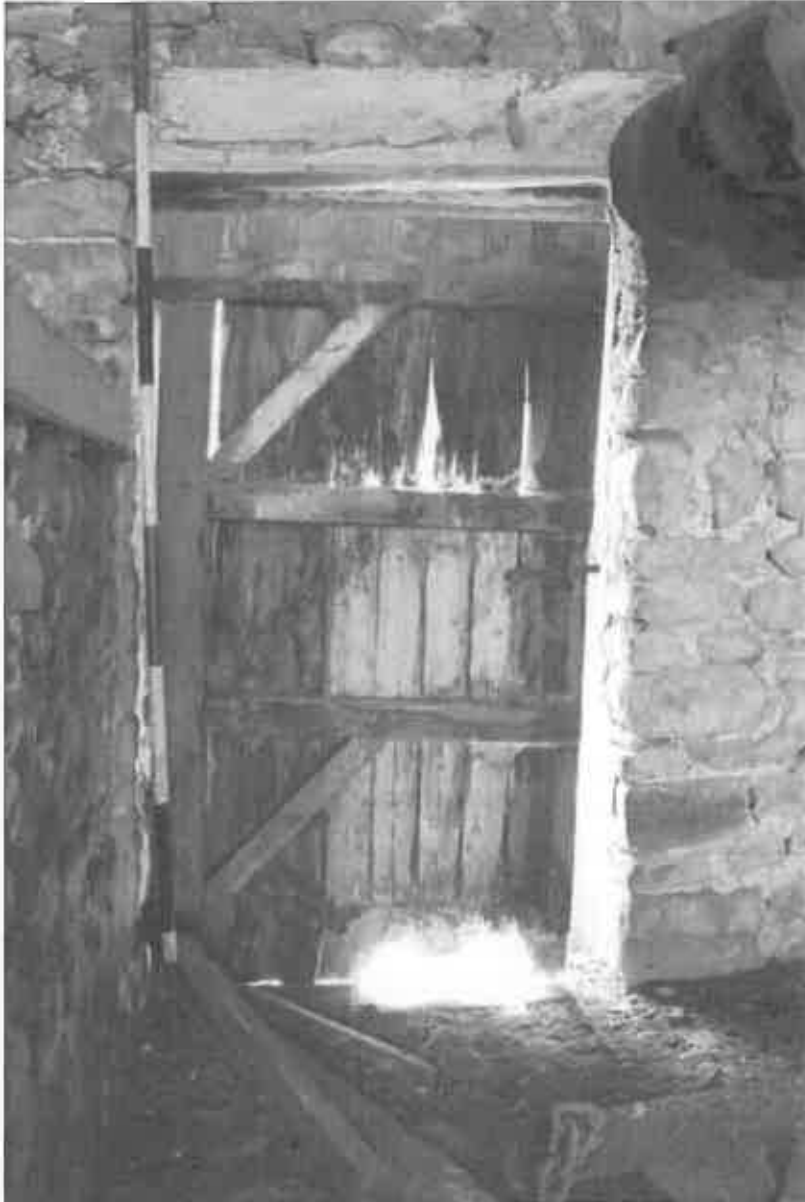
Figure 38 The doorway to the north west elevation.
