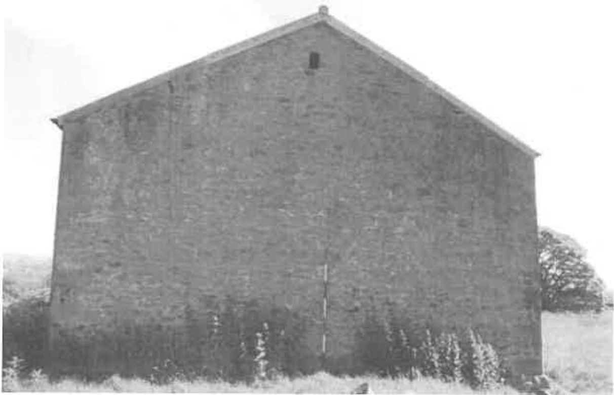
Figure 13 The north west gable elevation
