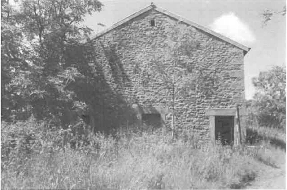
11 The south east gable end, with three ground level openings and the owl hole towards the ridge.
