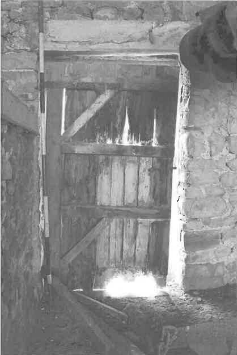
47 The door opening to the south west elevation, with the stone rebated jambs
