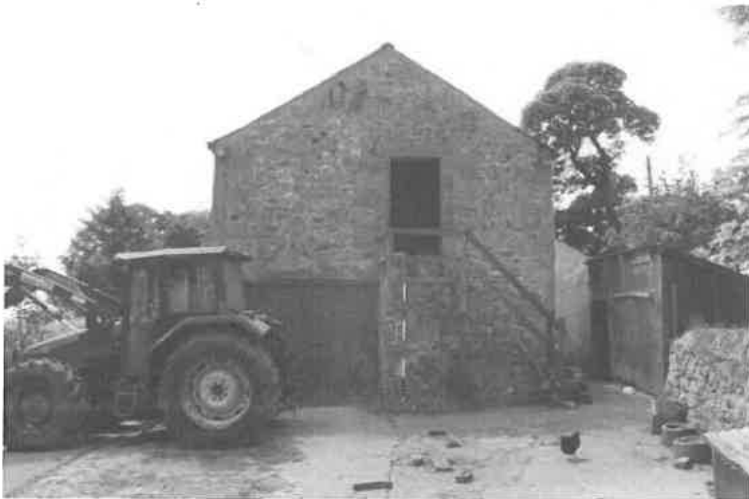
Figure.6 View of the first floor store at the north east end of the farmhouse
