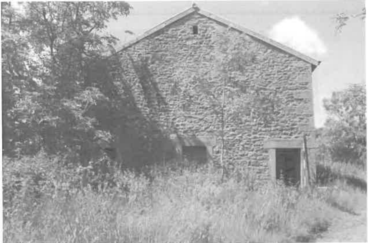
Figure 11 The south east gable end of the subject barn
