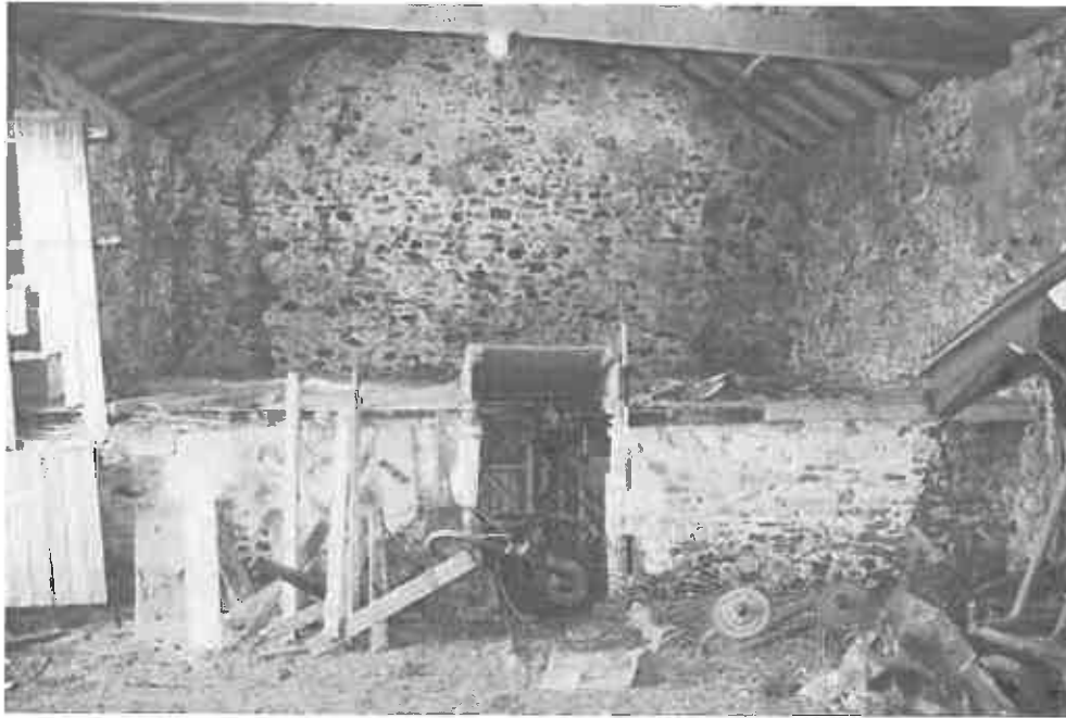
Figure 37 The partition wall and timber 'deck' to the south east elevation.
