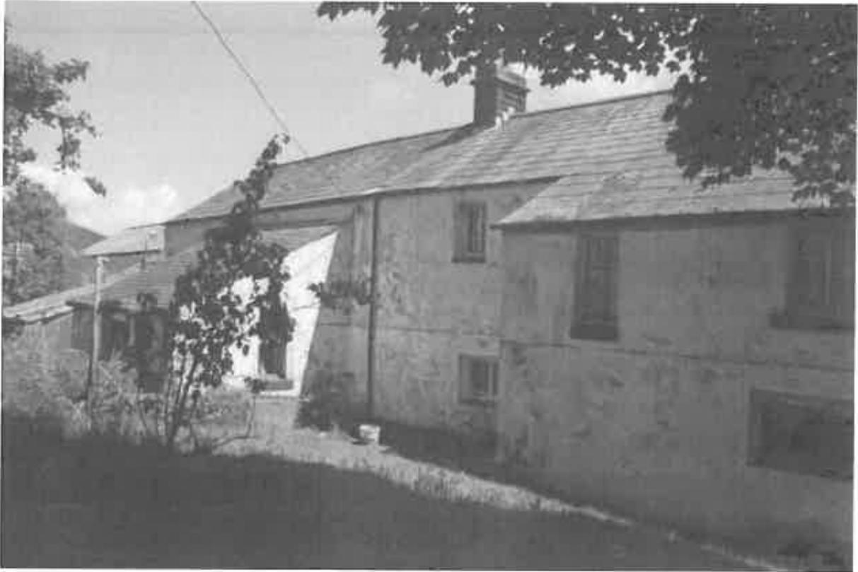
Figure 5 The rear of the farmhouse, with the outshut (or outshot) visible
