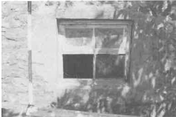
Figure 27 The window to the south west elevation.
