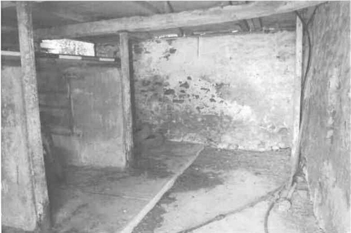
55 A view across the shippon with the concrete floor, stepped up towards the stalls.
