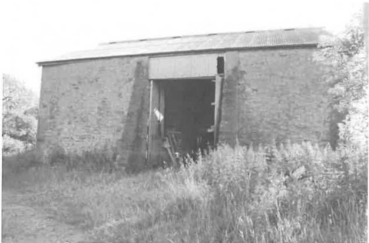
Figure 10 The subject barn as viewed from the north east.
