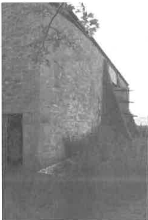
Figure 23 A view along the north east elevation showing the quoin detail to the corner.
