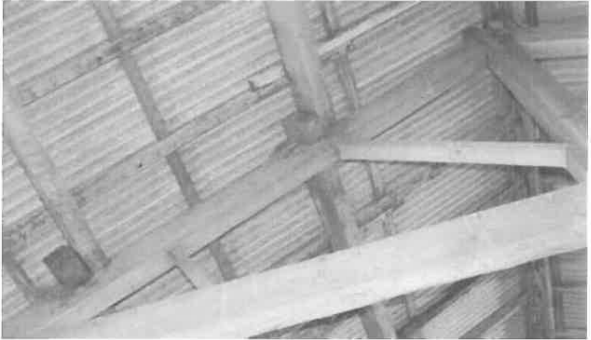
52 The staggered purlins to the north east roof pitch.
