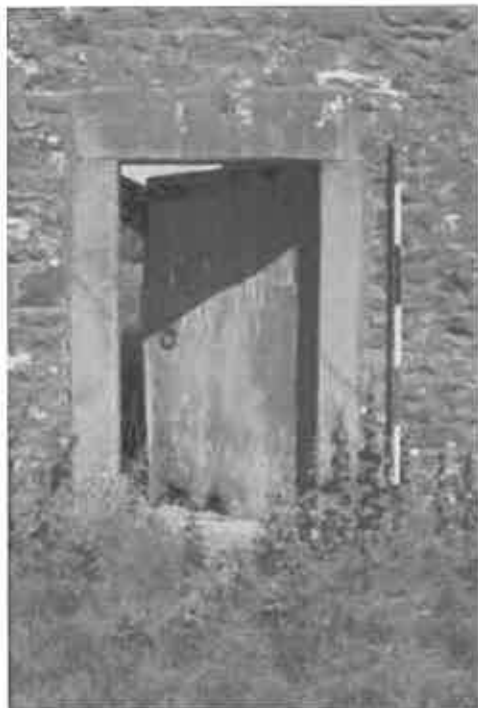
Figure 28 The doorway to the south west elevation.
