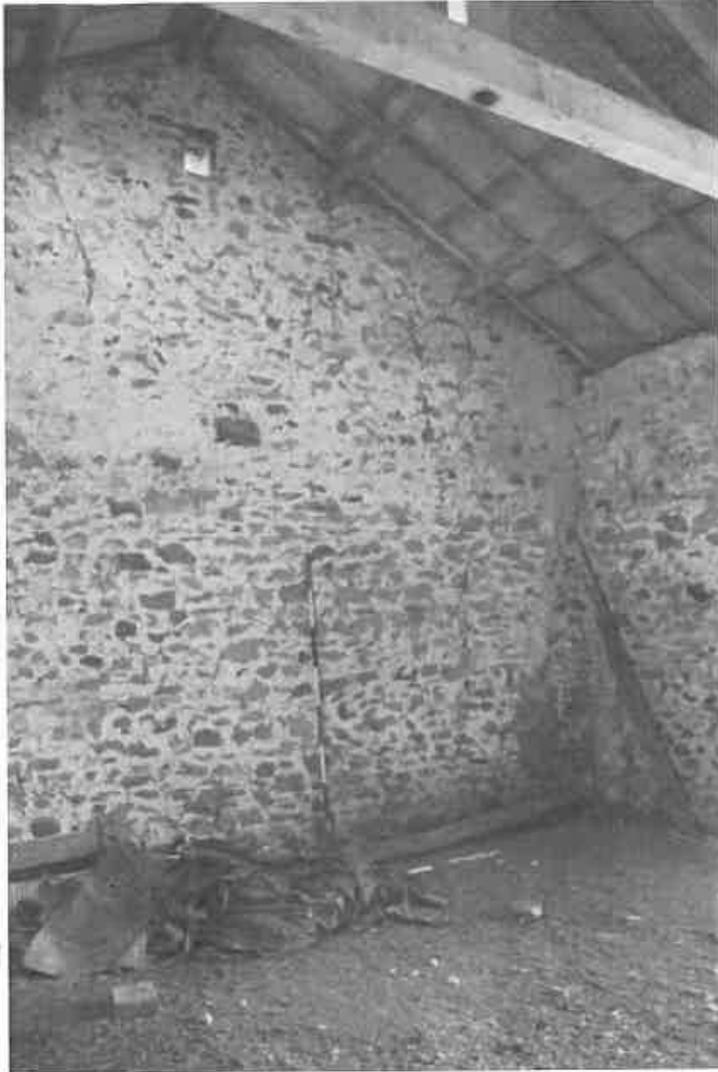
33 The internal corner to the north west and north east elevation.
