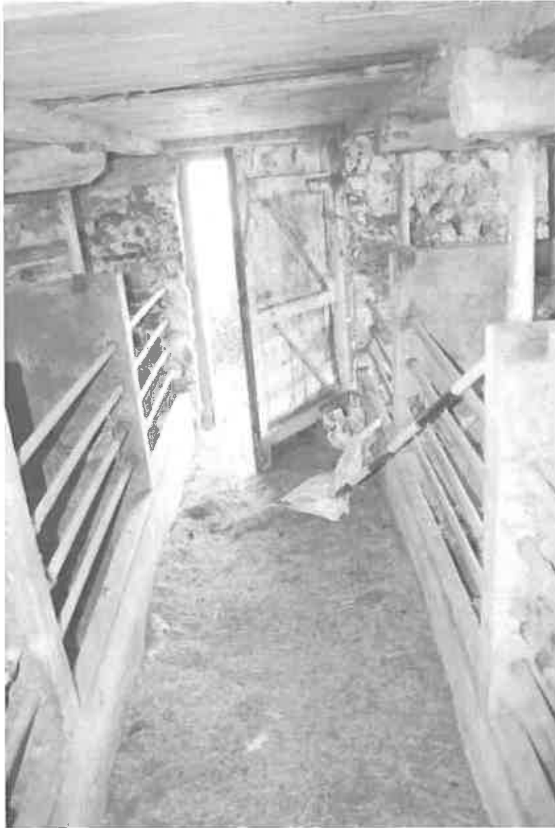
53 The central passage as viewed from the main barn area. The low level concrete back panels to the stalls, railings and the concrete floor are visible, along with the ends of the supporting beams.
