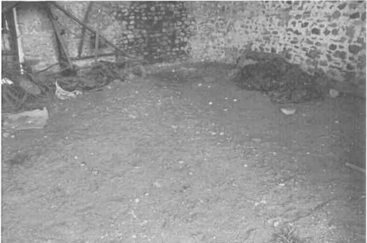
31 The compacted earth floor to the main area of the barn.
