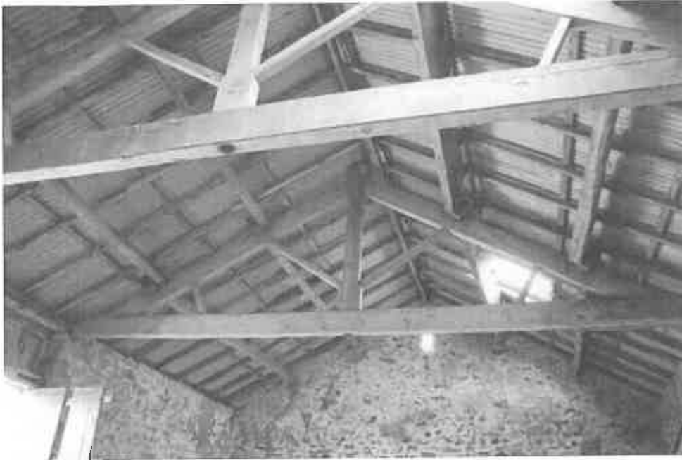
Figure 40 The roof structure, with staggered back purlins.
