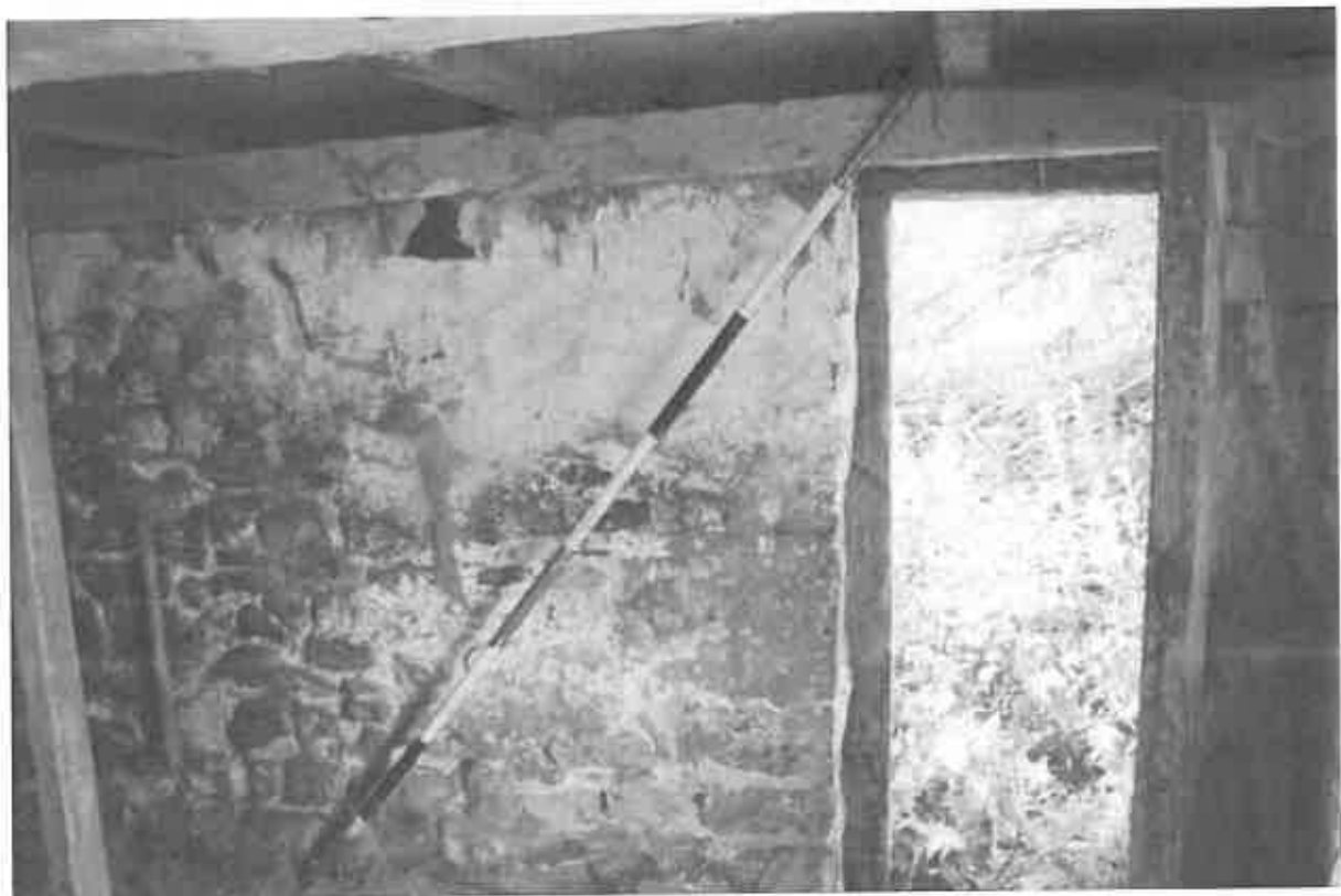
69 The stone 'corbel' to the gable elevation.
