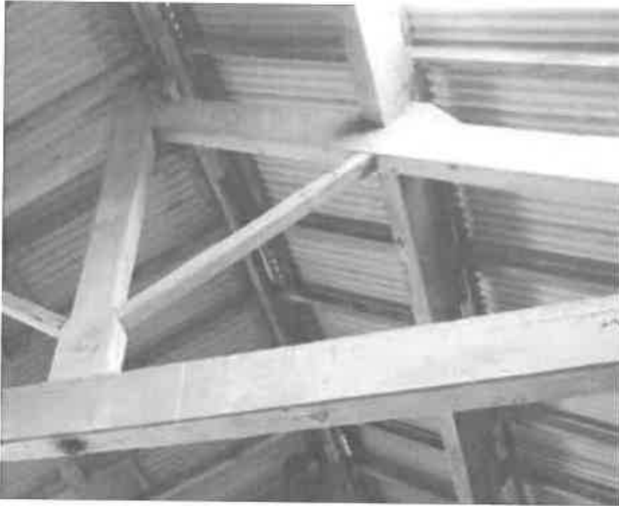
50 The cleated purlin to the principal rafter.
