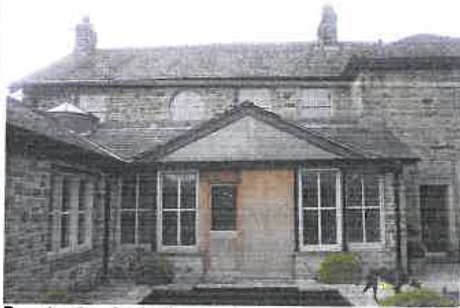
Rear elevation showing the extension
