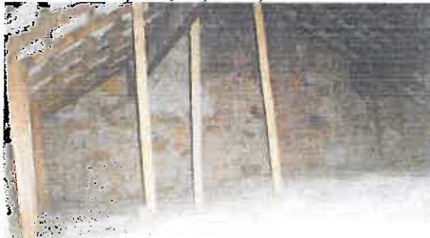
Internal south east gable
