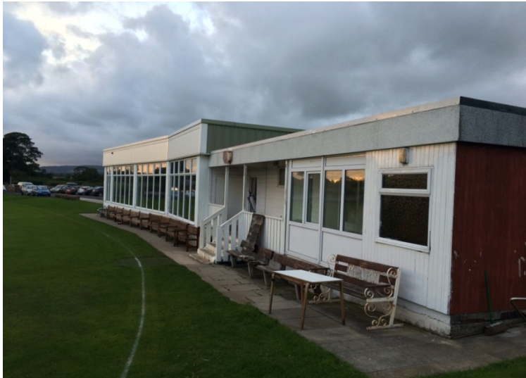
Plate 3.1 showing the exterior construction of the cricket pavilion
