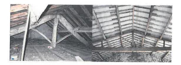
Roofing is in generally good condition although some gaps particularly in ridge tiles is present.
