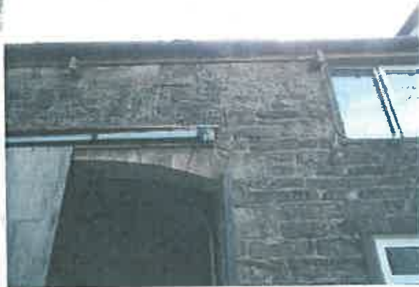
West wall showing part remove door support West wall showing movement to stones above door
