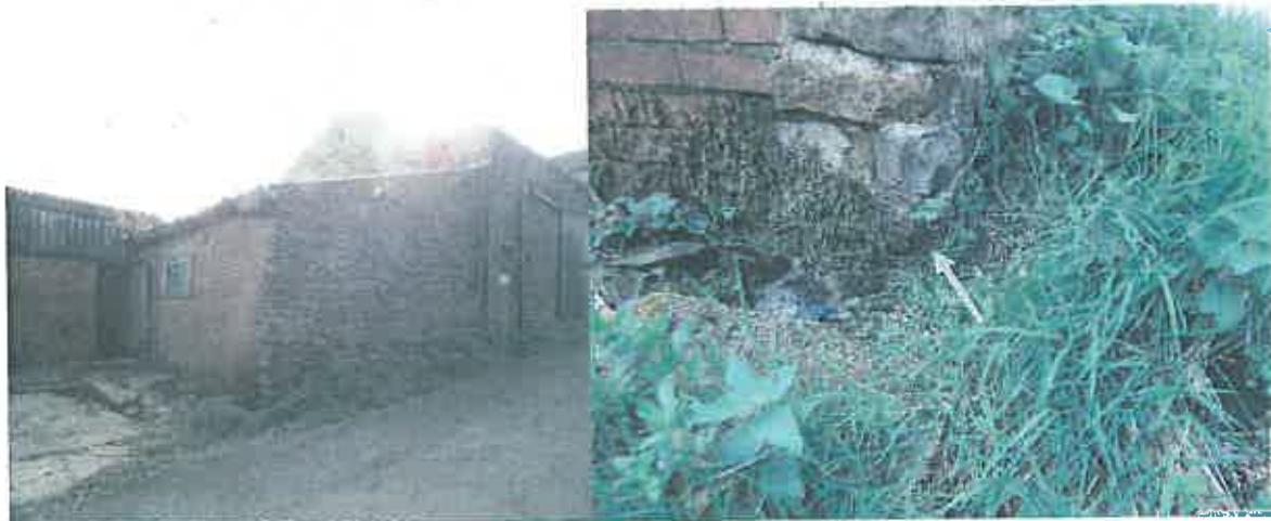
Milking parlour looking at north and west walls, Corner of wall has no under support.
