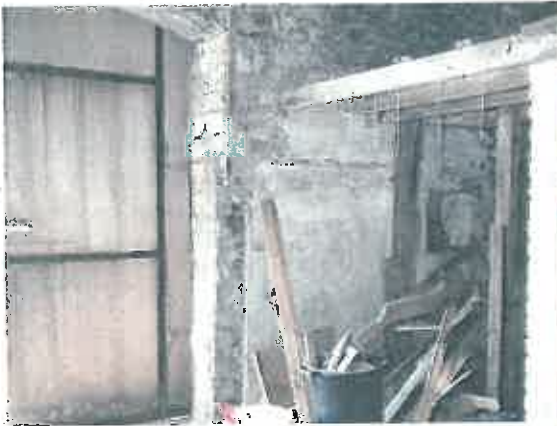
West wall showing part remove door support West wall showing movement to stones above door
