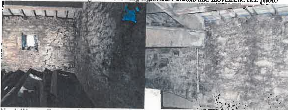
West wall mid section cracks next to kingpost
