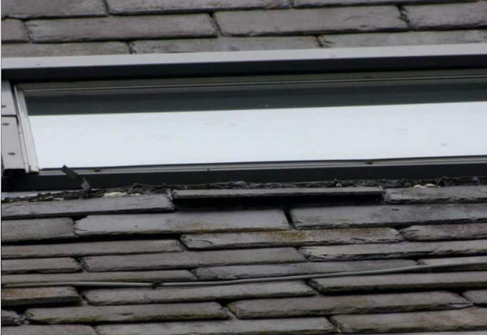
Example of lifted lead flashing
