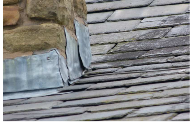
Example of lifted lead flashing
