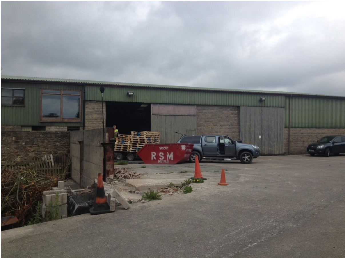
Figure 2: Picture of monitoring position viewed from the nearest noise sensitive receptor
