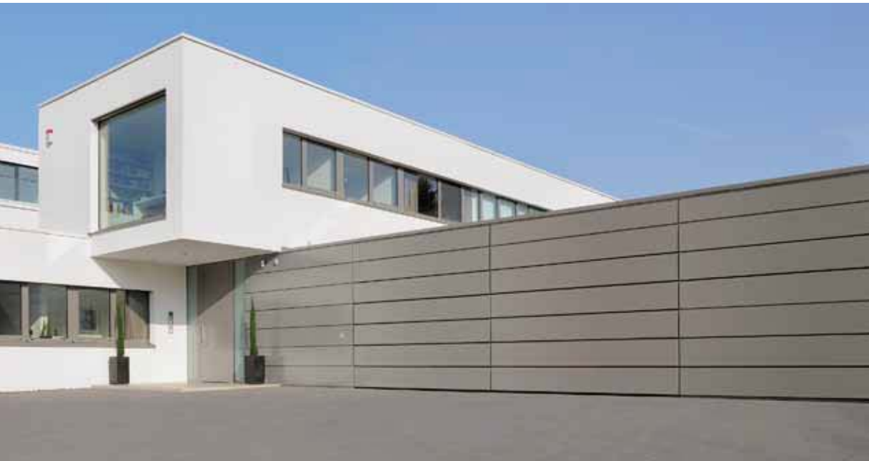
On-site cladding with aluminium compound board
