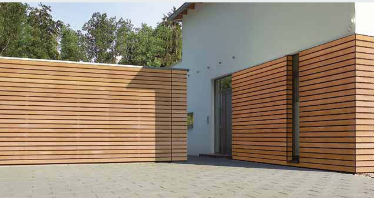
On-site cladding with timber panels
