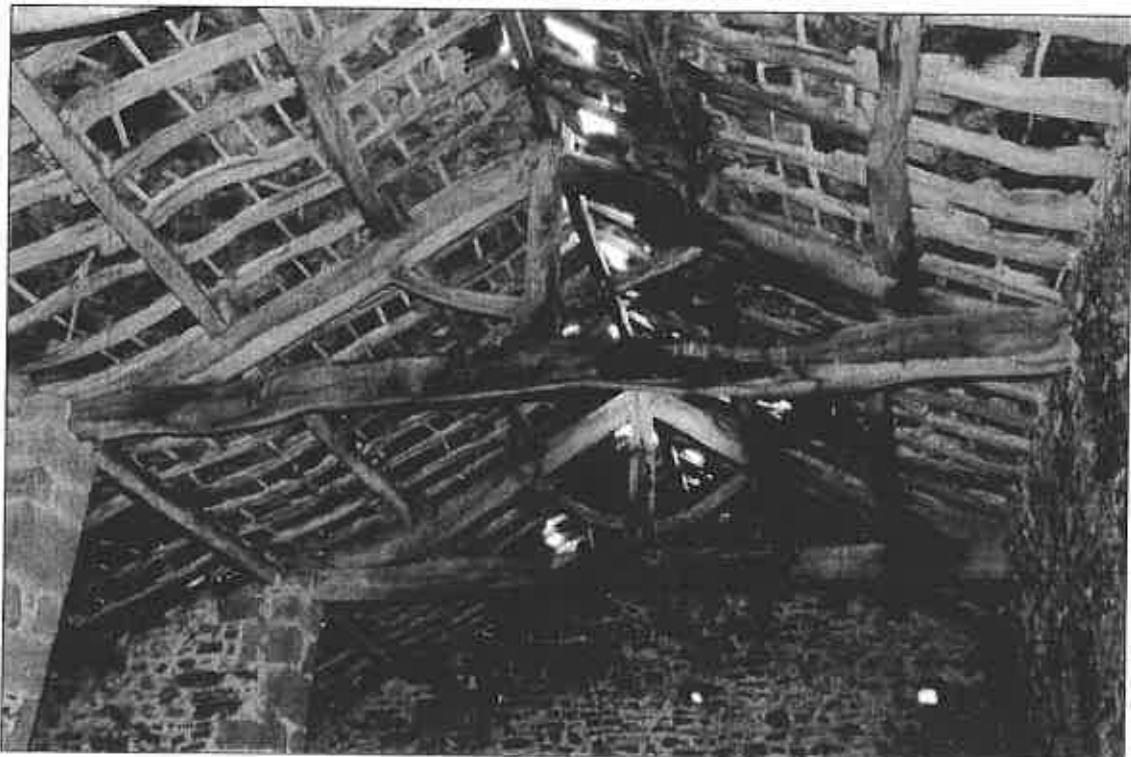
Photo 4: distinctive roof structure
