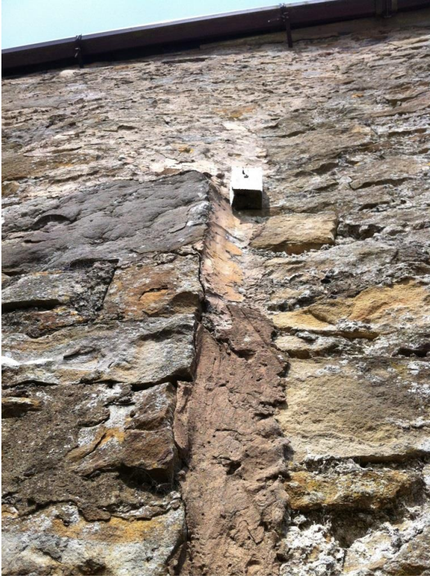
Photo 2: Inward lean to the rear elevation
