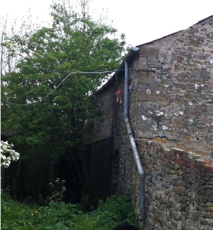
Photo 2: Inward lean to the rear elevation
