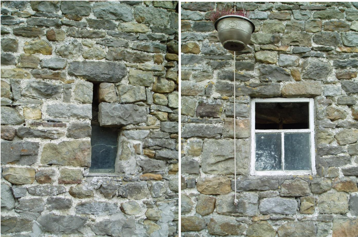
Breathing holes modified to create small windows.
