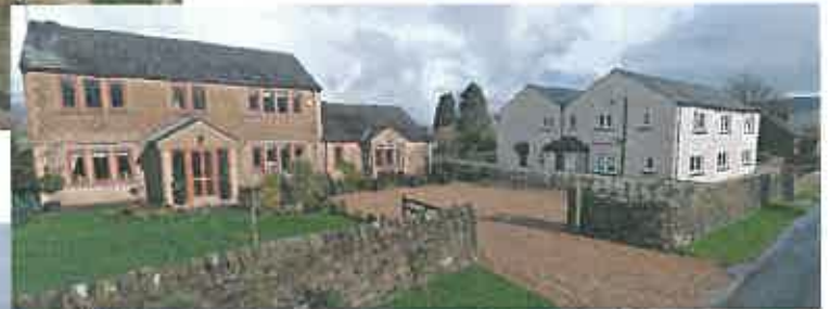
Fig 3– Maycroft House stone effect finish and the neighbouring property with a rendered finish
