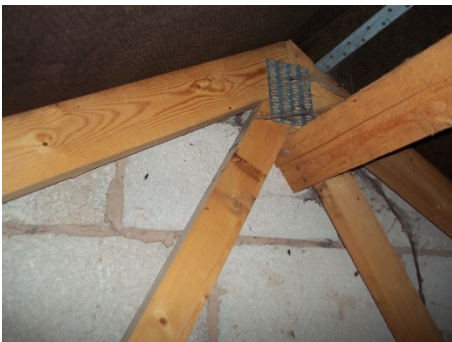
Figure 4: Roof void (west gable apex)
