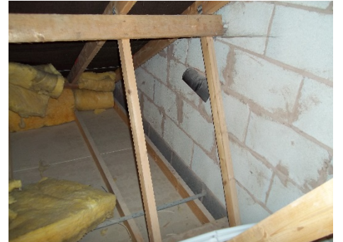
Figure 6: gable end wall, east elevation
