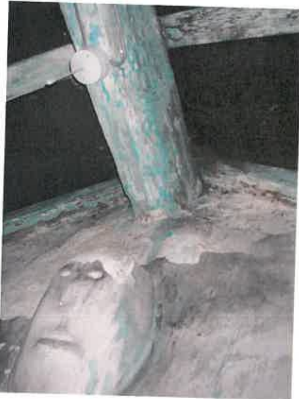
Fig 5 Inside the main loft.
