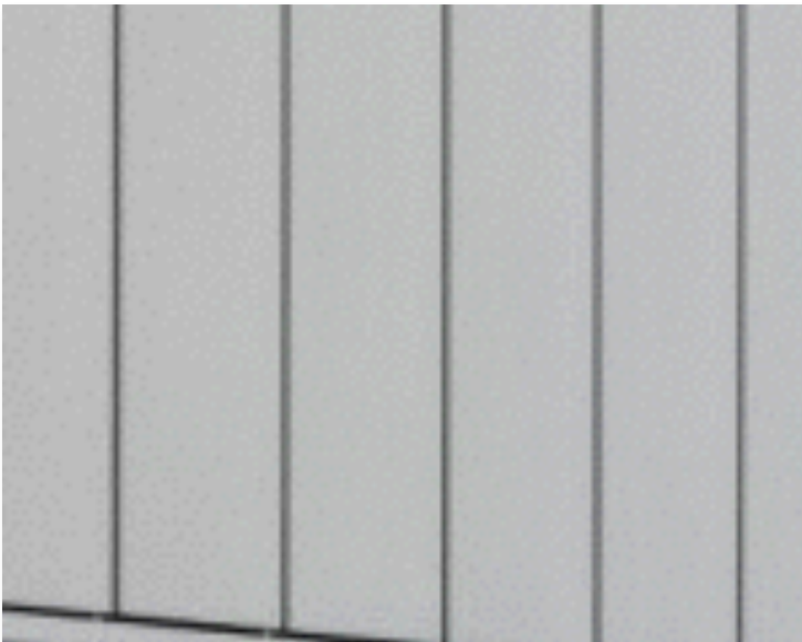
Cladding Standing Seam Zinc Cladding
