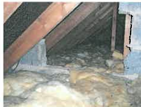
Figure 5: main roof void
