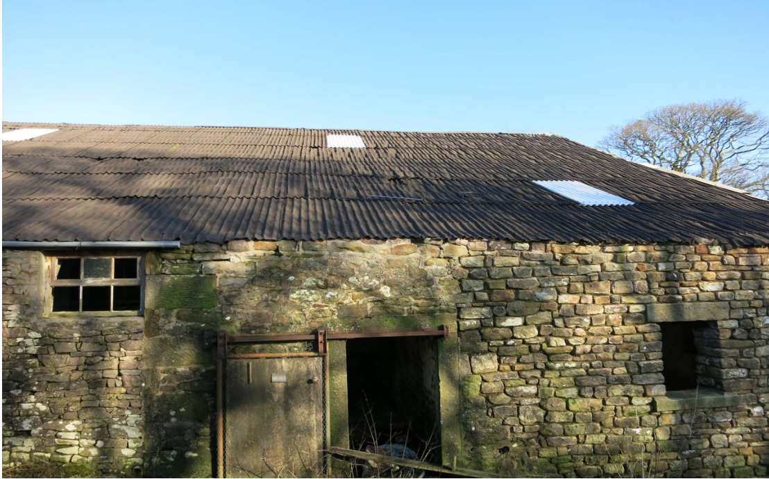
Exposed roofing underfelt with slates removed.
