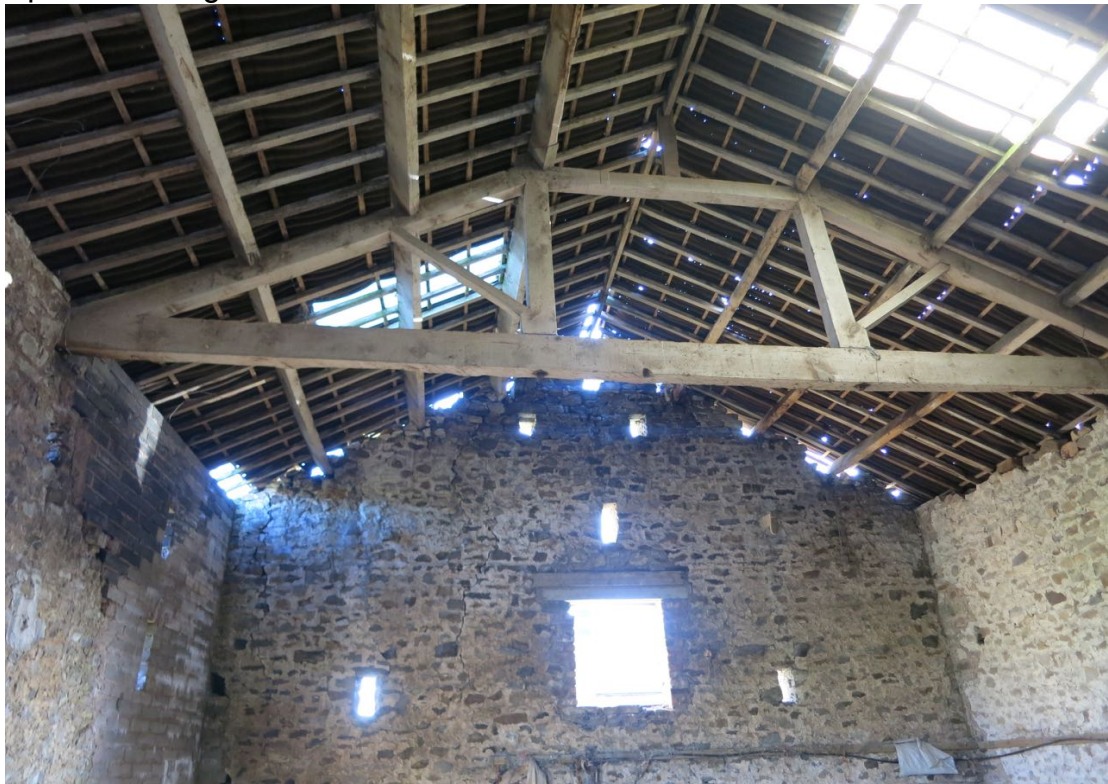
Considerable light penetration internally
