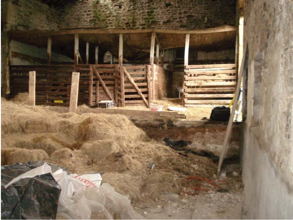
Plate 25 – Ground floor viewed from south-east corner
