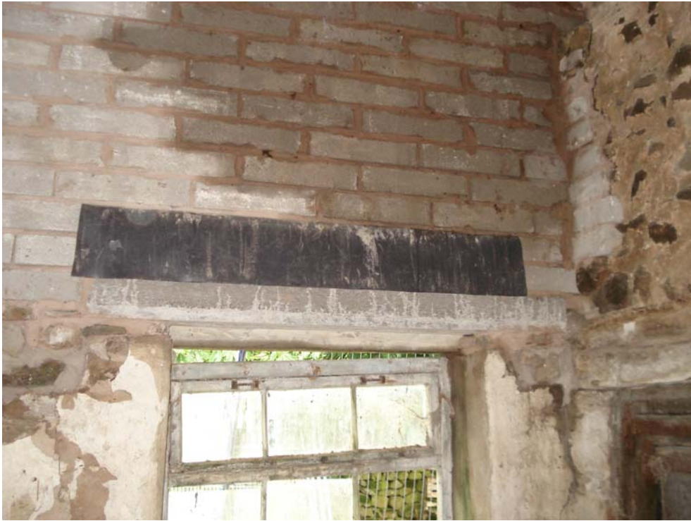
Plate 21 – Pre-stressed concrete lintel replacement
