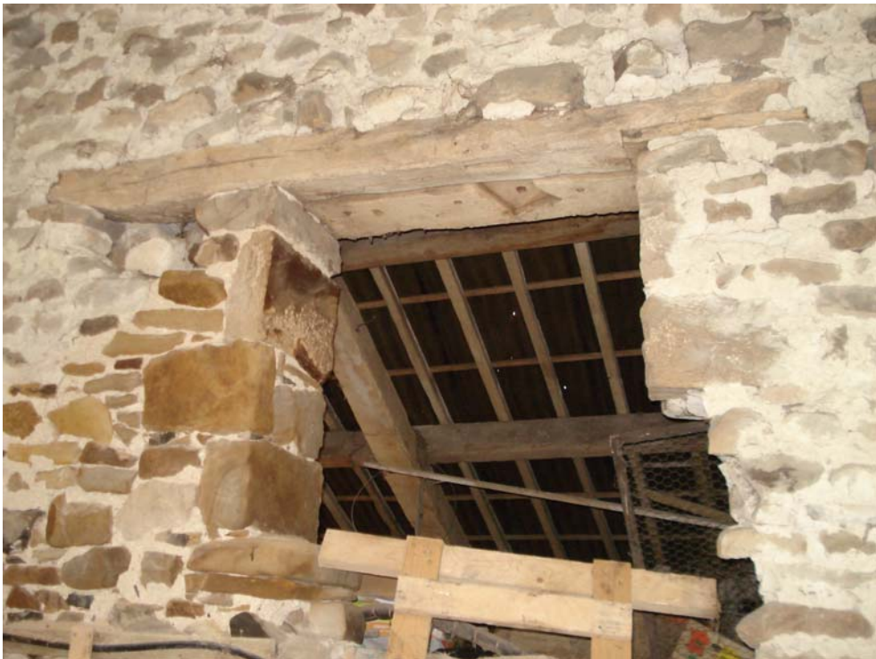
Plate 26 – Opening within rear elevation of barn to roof void of Shippon
