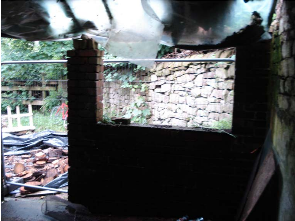
Plate 37 – Re-built brickwork elevation
