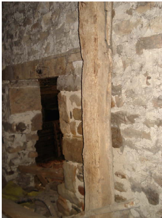
Plate 28 – Vertical post of mono pitch truss
