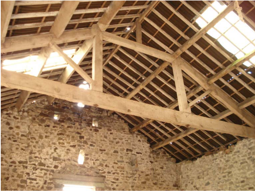
Plate 15 – Main Barn Roof
