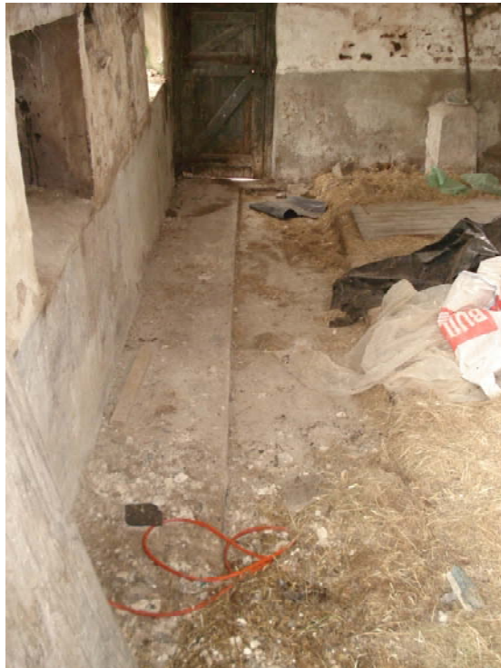
Plate 24 – Lower lying concrete ground bearing slab
