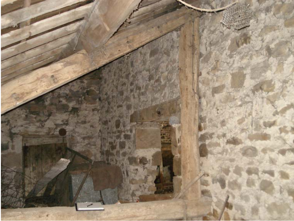
Plate 27 – Shippon roof (truss in foreground)
