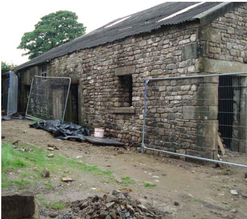
Plate 12 – Rear (west facing) Elevation
