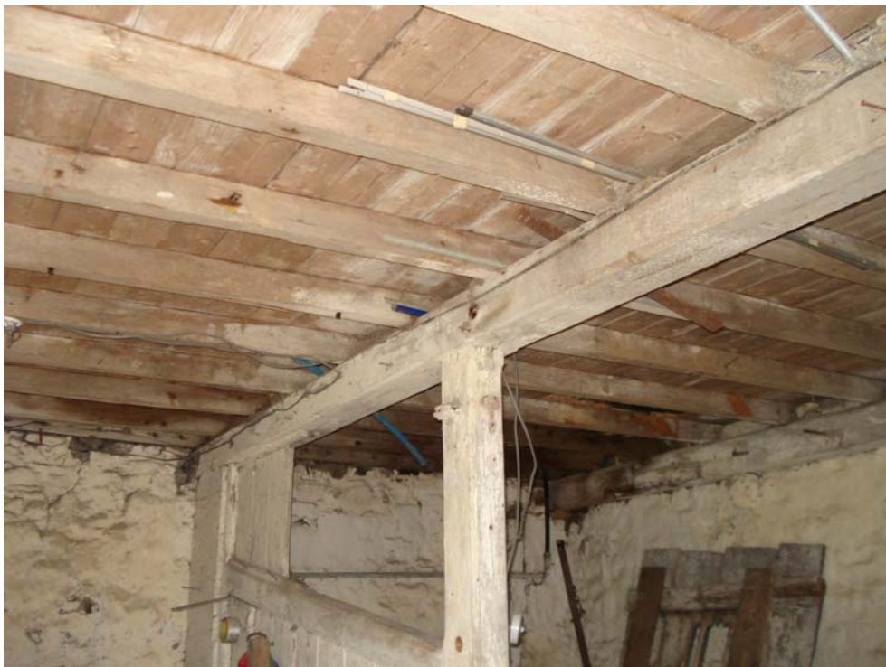
Plate 32 – 1 st floor joists supported on stall partition
