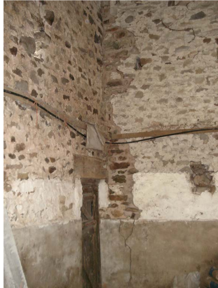
Plate 20 – South gable / Rear barn junction
