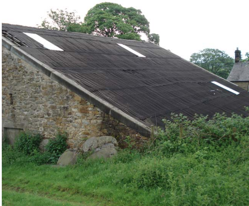
Plate 2 – Undulating roof finishes to rear pitch
