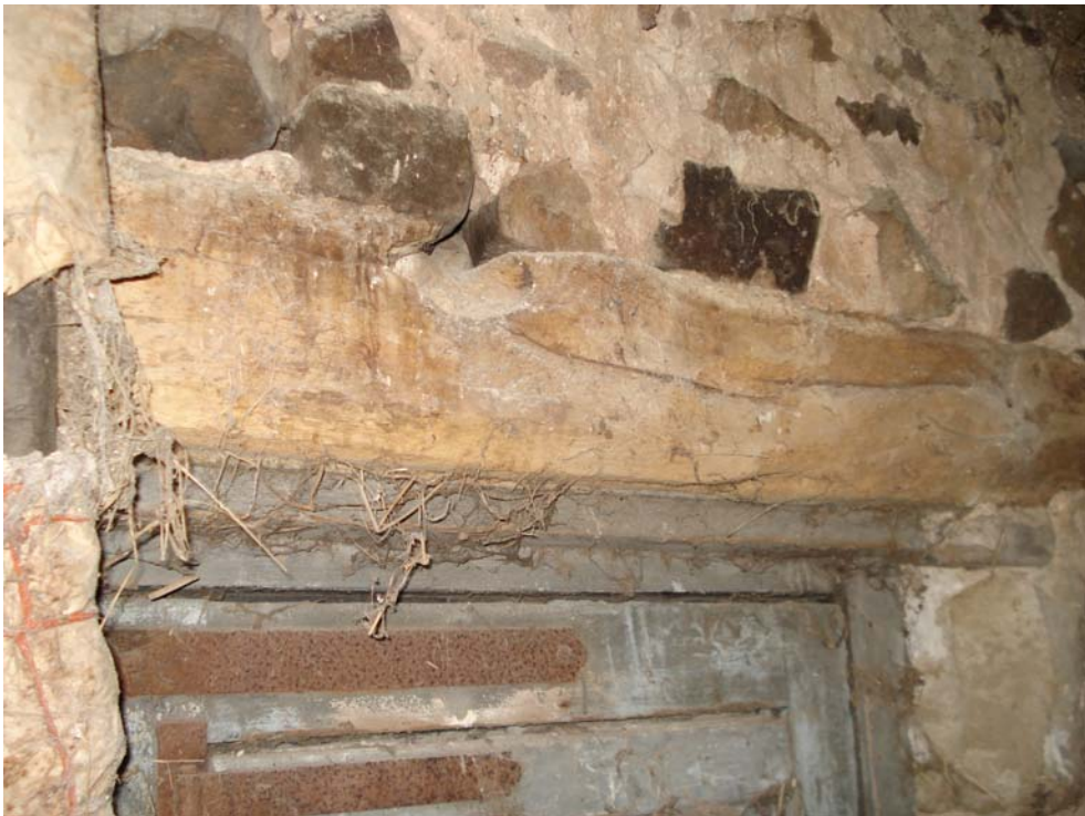
Plate 22 – Existing timber lintel (Barn – internal)
