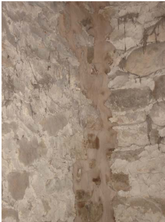
Plate 34 – Butt joint at Shippon / Barn
