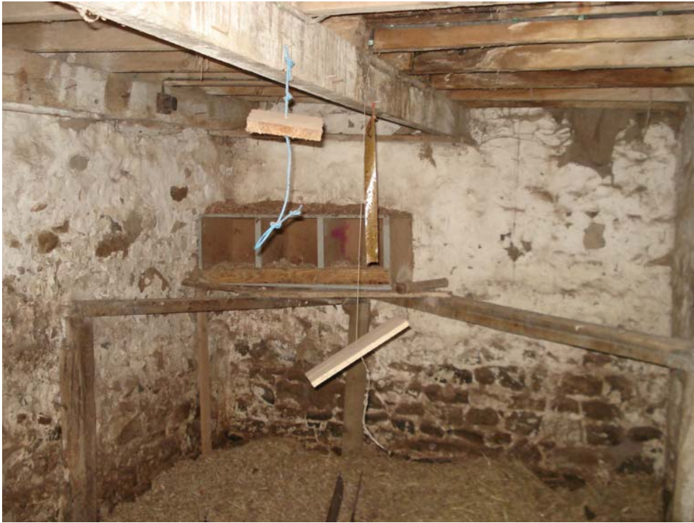
Plate 33 – 1 st floor supporting beam
