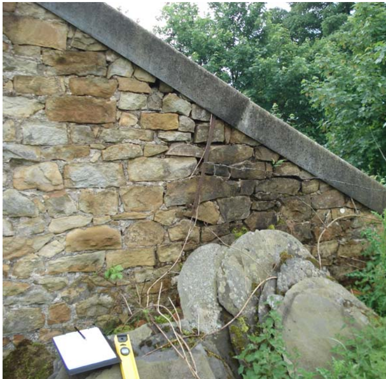
Plate 4 – Damp 'staining'
