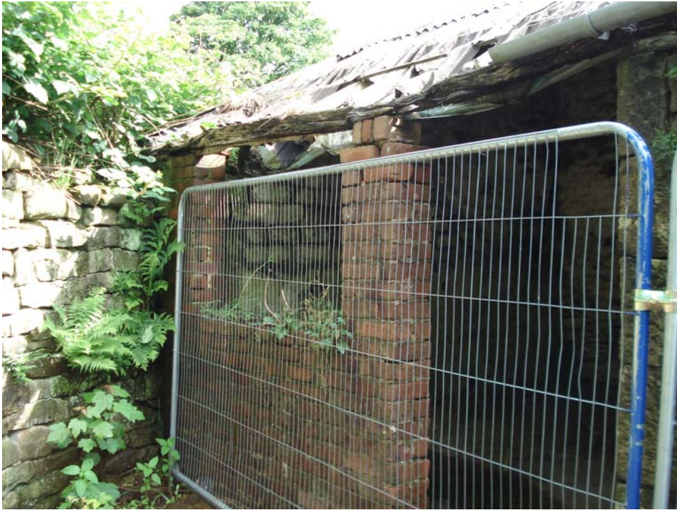
Plate 13 – Rebuilt brick facade adjacent to North Gable
