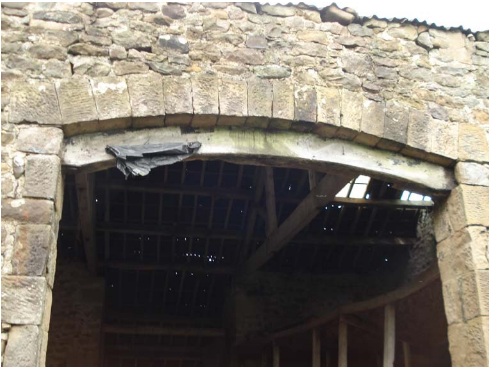
Plate 6 – Timber lintel beneath masonry arch
