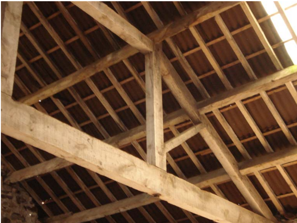
Plate 16 – Main Barn Roof
