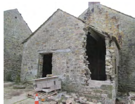
Images showing collapse of the North East corner during the underpinning works.
