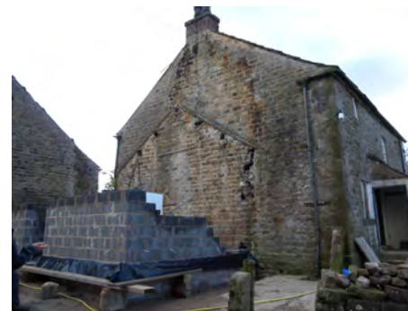
Image showing extent of rebuild to the single storey outbuilding
