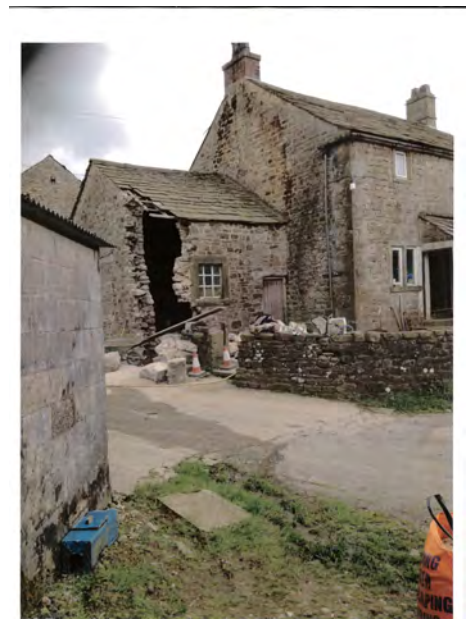
Images showing collapse of the North East corner during the underpinning works.
