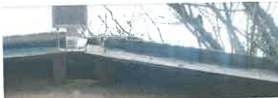
Shed 1- Corrugated fibre sheet over timber purlins
