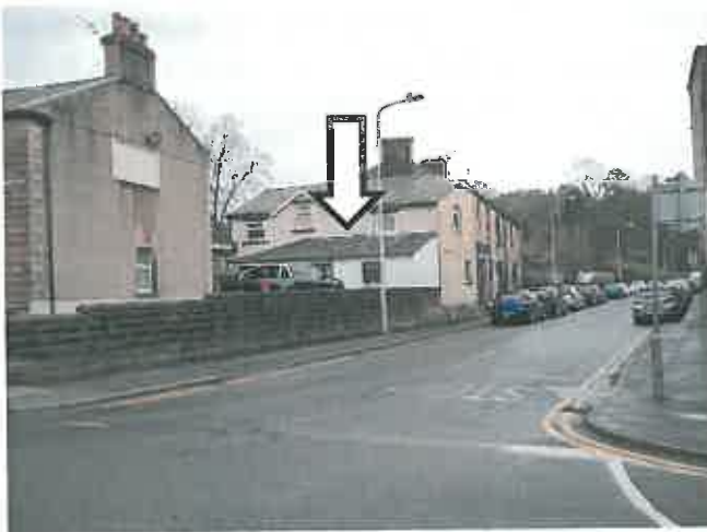
Figure 9: View north along Woone Lane showing premises.
