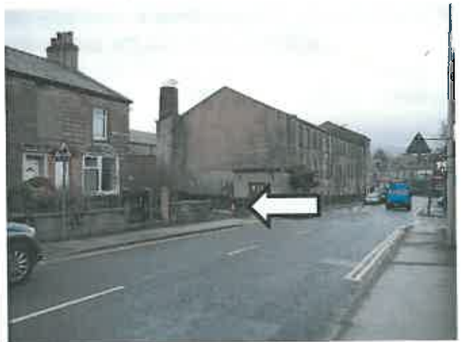
Figure 10: View east along Eshton Terrace to access
