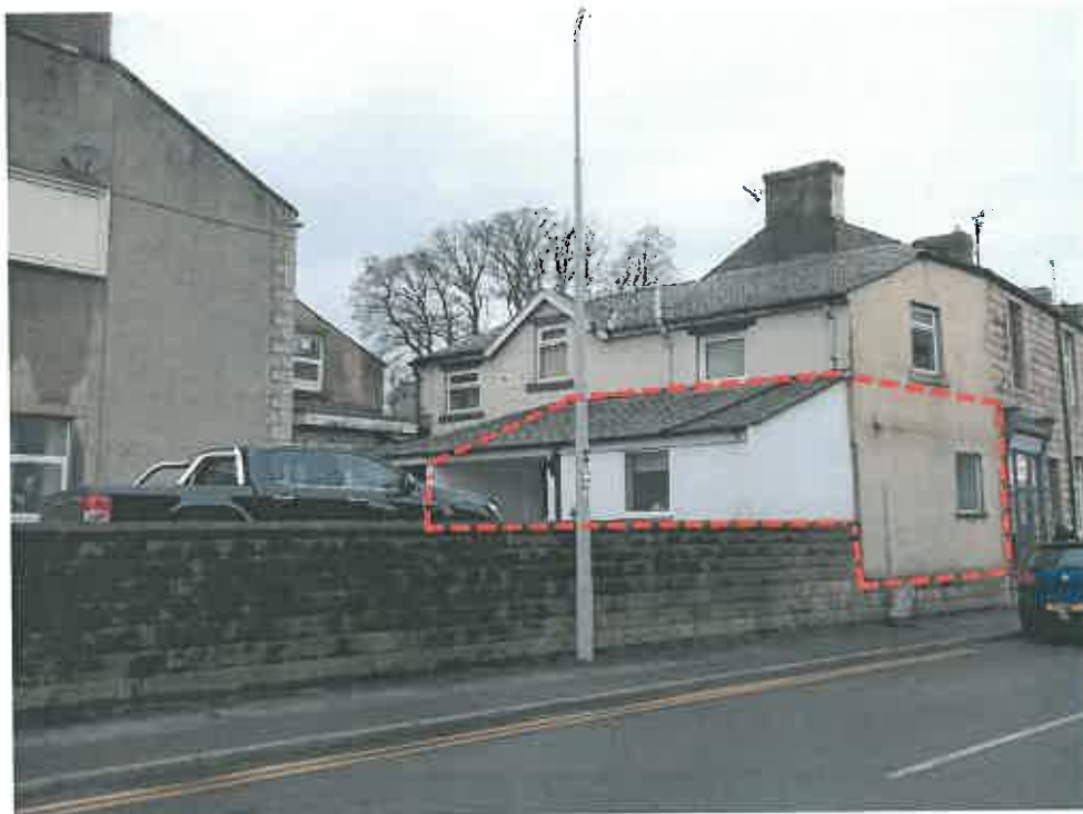
Figure 1: No. 4 Eshton Terrace
