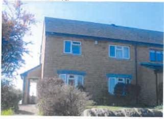
The property is a semi detached house built in 1996. It has a lean-to porch to the side and a single storey lean to across the rear elevation of the property. Part of the rear lean- to is a garden room with a plastic roof.
