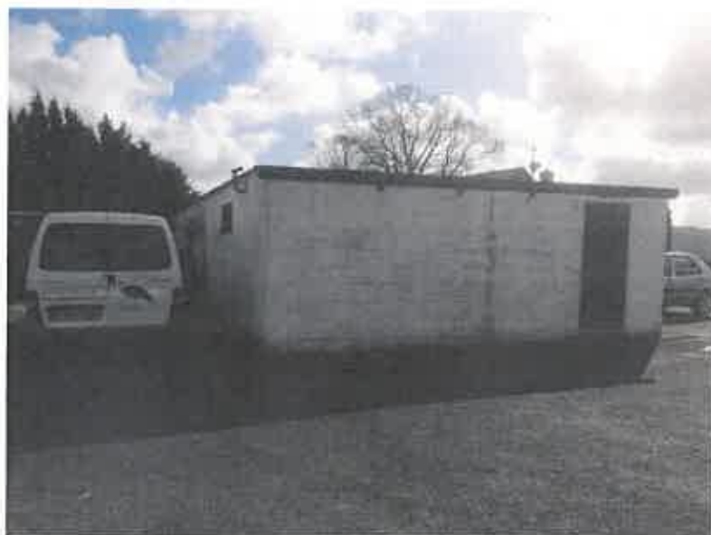
Side (west) elevation of existing store
