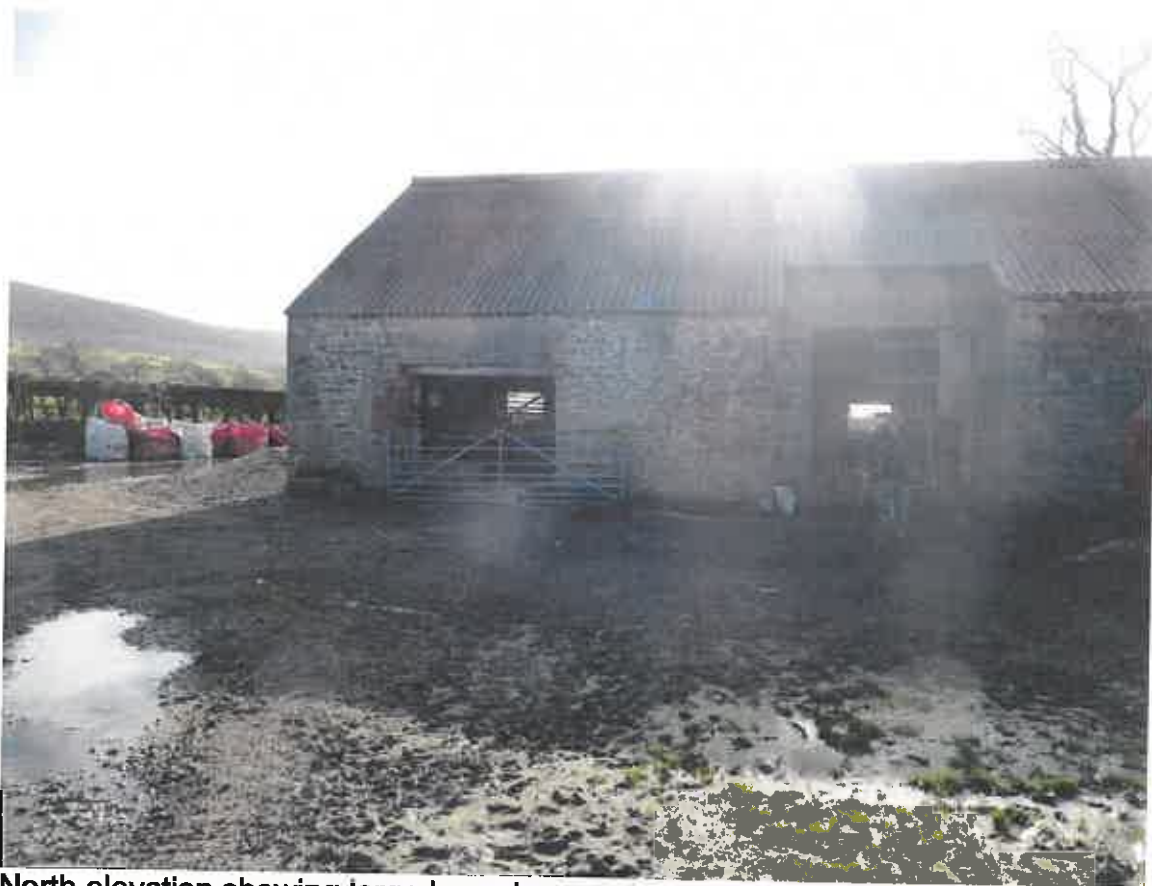
North elevation showing large barn door.
