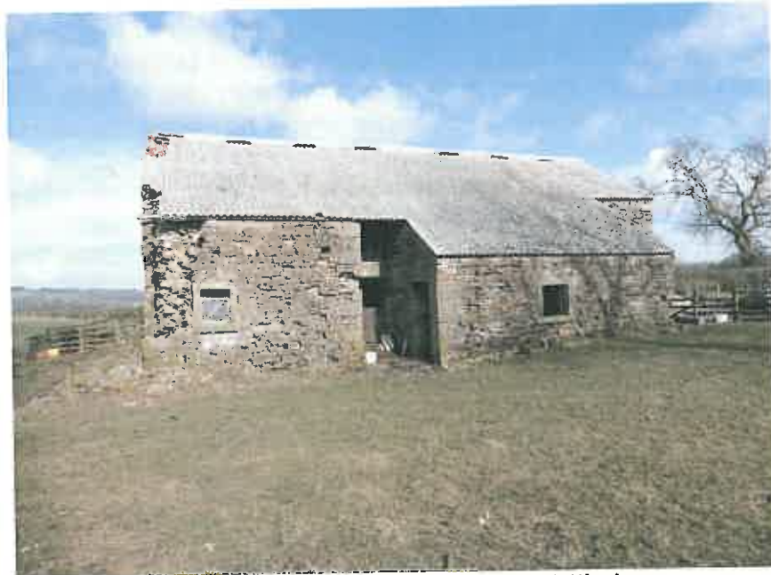
South elevation showing lean to cattle byre
