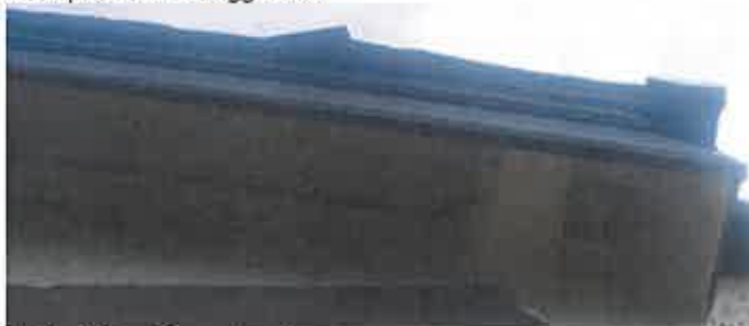
Underside of Barge boards
