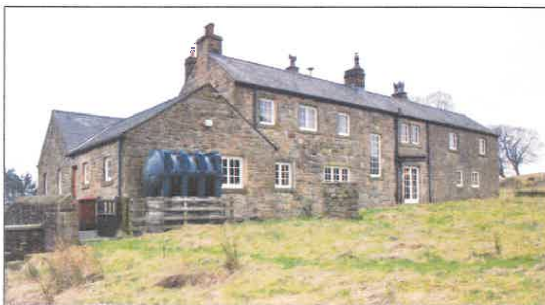
Rear view of the house
