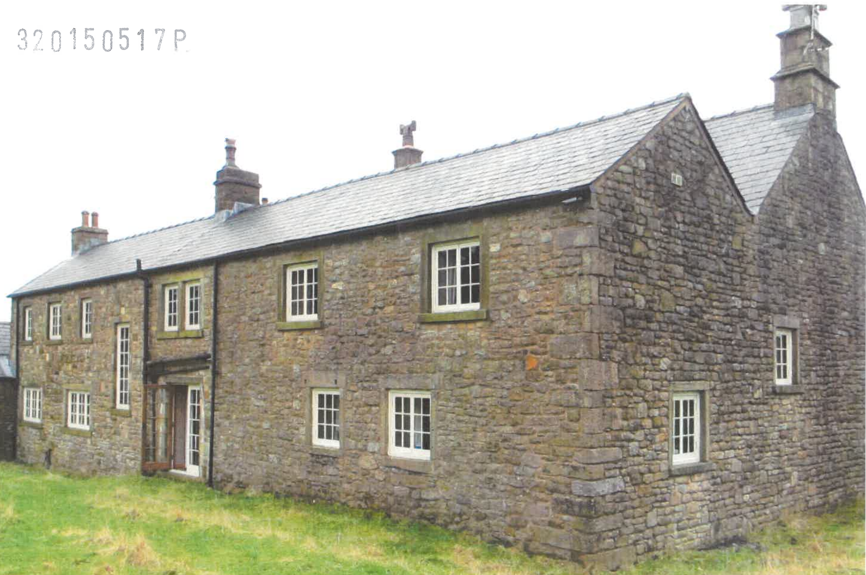
proposed extension rear of Wolfen Hall. chipping
